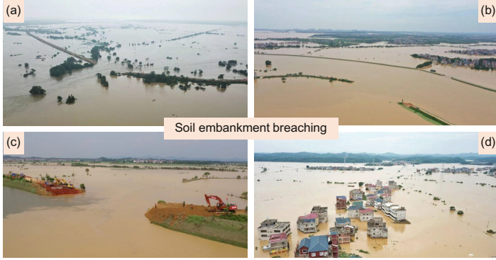
Fig. 2. Typical events of embankment breaching due to continuous heavy rainfall taken place in the Poyang Lake regions of China in July 2020 (Chen 2020).
