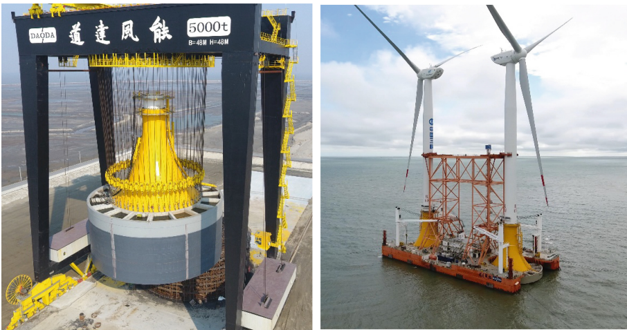
(a) Hybrid mono-bucket foundation
