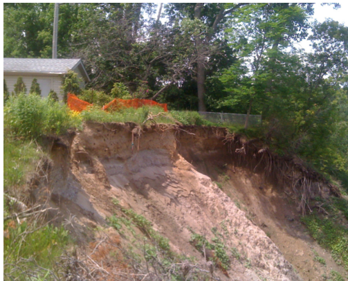
Fig. 5. Groundwater seeping out from sandy soil was observed at project site (picture taken by Ron Xia on June 11, 2015).
