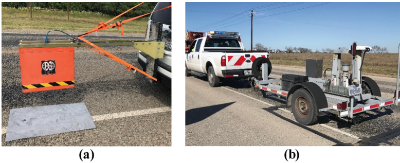
Fig. 8. Non-destructive testing in Texas overload corridors (a) GPR testing, and (b) FWD testing.
