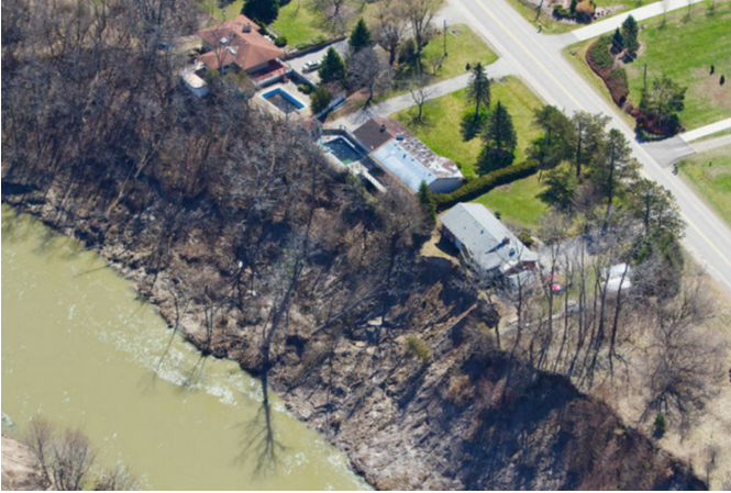
Fig. 3. Three homes on Adelaide Road are close to falling into the Thames River (Picture taking on April 17, 2013 by Mike Hensen 2013).
