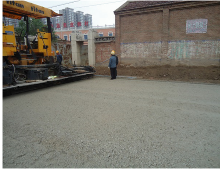
Fig. 1. Paving GBSB
