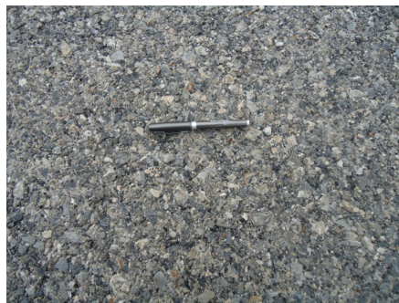
Fig. 3. The effect of GBSB after rolling and forming
