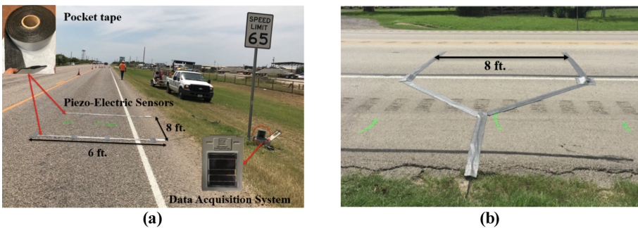
Fig. 3. Deployment of the P-WIM devices in the field, (a) Typical P-WIM system setup, (b) Arrangement of installed piezo-electric sensors.
