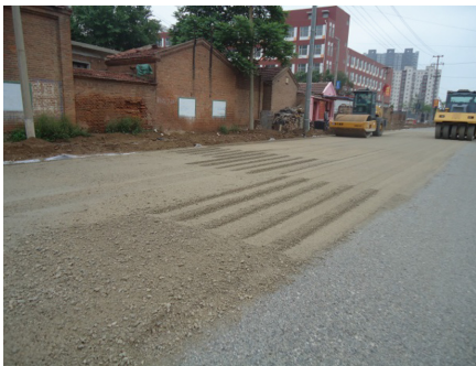
Fig. 2. Rolling of graded gravel base
