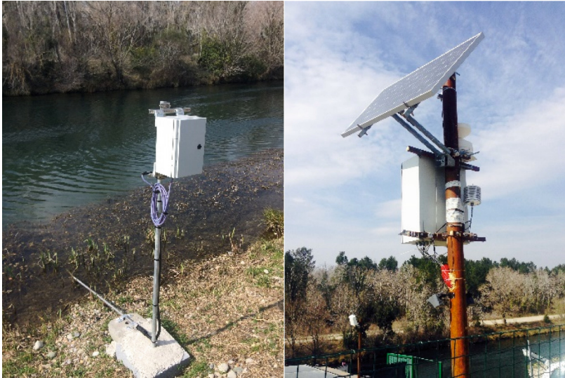
Fig. 3. THM logger on the downside of the embankment (left) solar system and metrological sensor (right)
