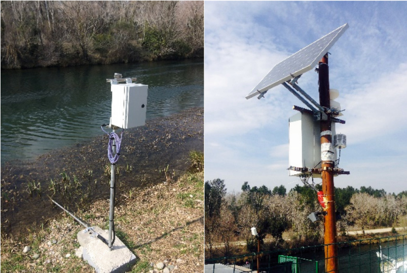
Fig. 3. THM logger on the downside of the embankment (left) solar system and metrological sensor (right)
