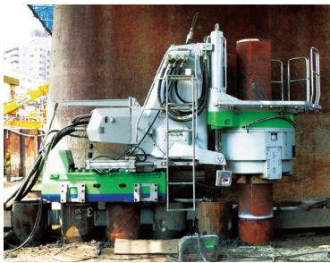
a) Self-walking system (as known as SILENT PILER)
