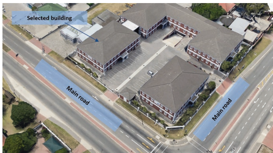
Fig. 12.1 Selected office building
