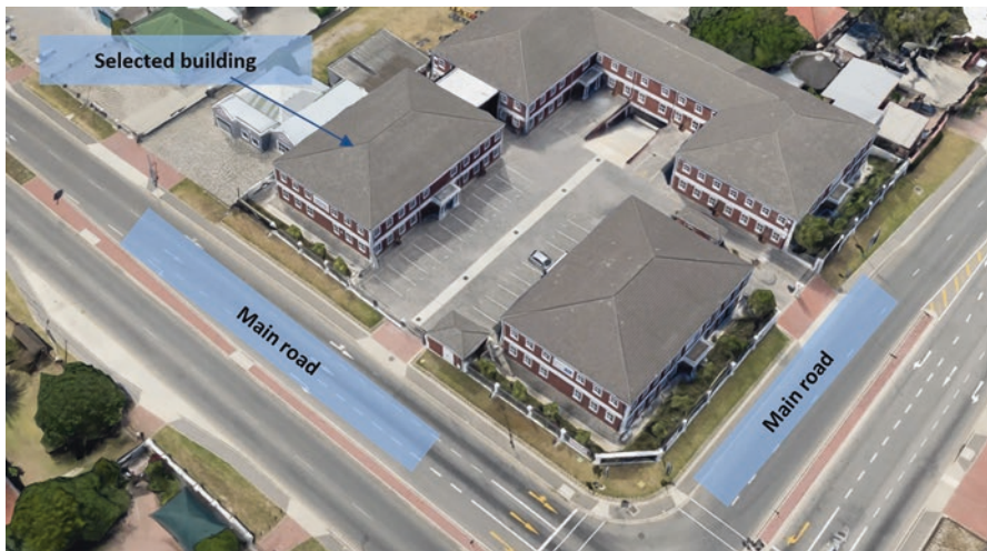
Fig. 12.1 Selected office building
