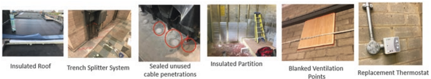
Fig. 5.4 Installed interventions pictured
