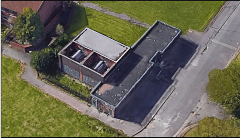
Fig. 5.1 Pendleton Primary Substation
