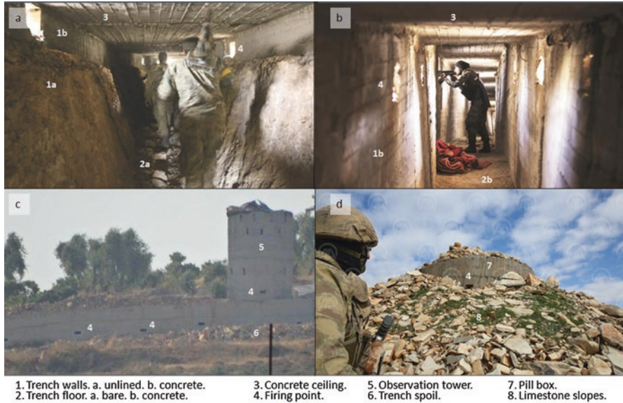
Fig. 17.6 (a) Unlined Syrian Kurdish defensive trench in chalky limestone with a rock floor and reinforced concrete overhead protection. (Modified from Yeni Safak 2018a). (b) Syrian Kurdish CCHT with multiple firing points. (Modified from Yeni Safak 2018c). (c) View of Syrian Kurdish CCHT combined with an OT on Mount Bursaya. (Modified from Southfront.org 2018). (d) Syrian Kurdish pillbox at Mount Bursaya. (Modified from Prima News 2018)
