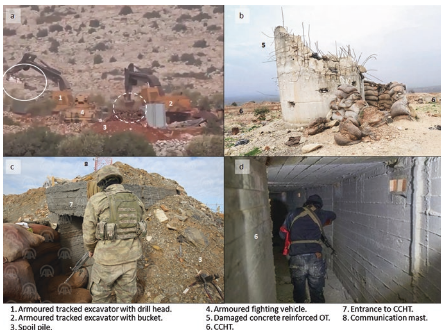
Fig. 17.10 (a) Trench excavated by TAF 10 November 2017 on a limestone slope using armoured tracked excavators. (Modified screenshot from https://www.youtube.com/watch?v=5UajSoNxMwI ). (b) Syrian Kurdish concrete reinforced cylindrical OT on Mount Sakarkaya destroyed by either an air or artillery strike, revealing the rebar mesh. (Modified from Yeni Safak 2018b). (c) Entrance to a Syrian Kurdish CCHT at Mt Bursaya captured by TAF and TFSA. (Modified from Prima News 2018). (d) TFSA fighter in a Syrian Kurdish CCHT at Mt Sakarkaya. (Modified from Daily News 2018a)
