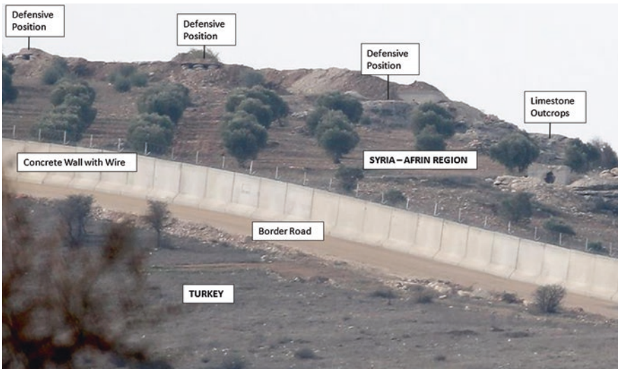
Fig. 17.4 View from the Turkish side of the border over a defensive wall to the Syrian side on 17 January 2018. Defensive positions constructed on the crest of the limestone ridge can be seen on the Syrian side. (Modified from Chohan 2018)
