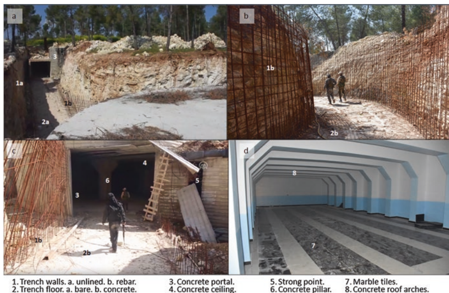
Fig. 17.7 (a–c) Entrances to Syrian Kurdish UGFs in the mountains around Afrin constructed in a chalky limestone. (a and c modified from NTV 2018, b modified from Syria Call 2018). (d) Room in a Syrian Kurdish UGF in the mountains around Afrin with 100-m tunnels. (Modified from Syria Call 2018).
