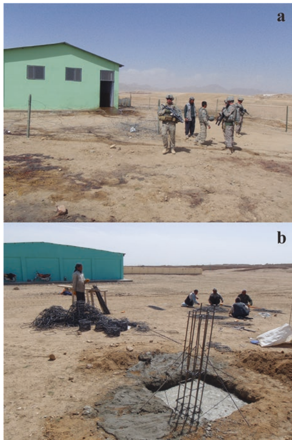
Fig. 14.4 Ground photographs of the Ghazni Agricultural Complex in March 2009. (a) This photo looks westerly at the recently built slaughterhouse (red arrow on Fig. 14.3); note the blood-stained ground (especially front left). (b) This photo is easterly facing showing the new foundation emplacement for the sales barn (yellow arrow on Fig. 14.3)
