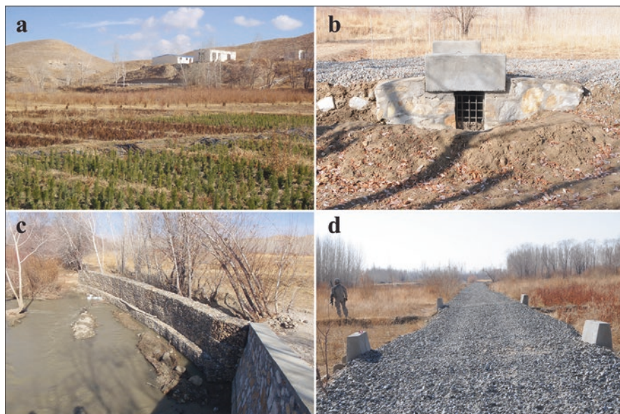
Fig. 14.8 Ground photographs of the Ghazni Demonstration Farm in December 2009. (a) View looking northeast across plotted conifer saplings with the classroom and cold storage in the distance (yellow arrow on Fig. 14.7a). Note the raveled drip-irrigation lines in the middle ground/right and the failure of approximately 50% of the saplings to take root. (b) An IED-resistant irrigation culvert. (c) A perspective view from the access bridge looking westerly at the recently emplaced gabion wall (white arrow on Fig. 14.7a). (d) Westerly view of the recently emplaced and graveled access road with four culvert abutments
