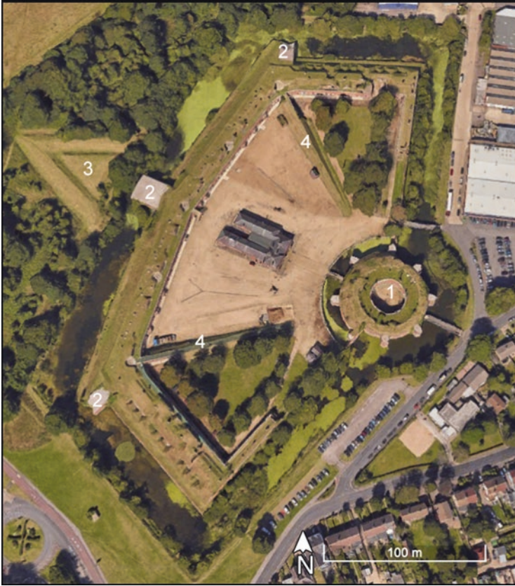
Fig. 3.13 Fort Brockhurst, Gosport Advanced Line. Note the round, Henrician-style keep (1), the caponiers in the moat (2), the earthen redan (3) and the ramps leading from the parade ground to the ramparts (4). (Modified from Google Earth Pro; image Landsat/Copernicus 2020)
