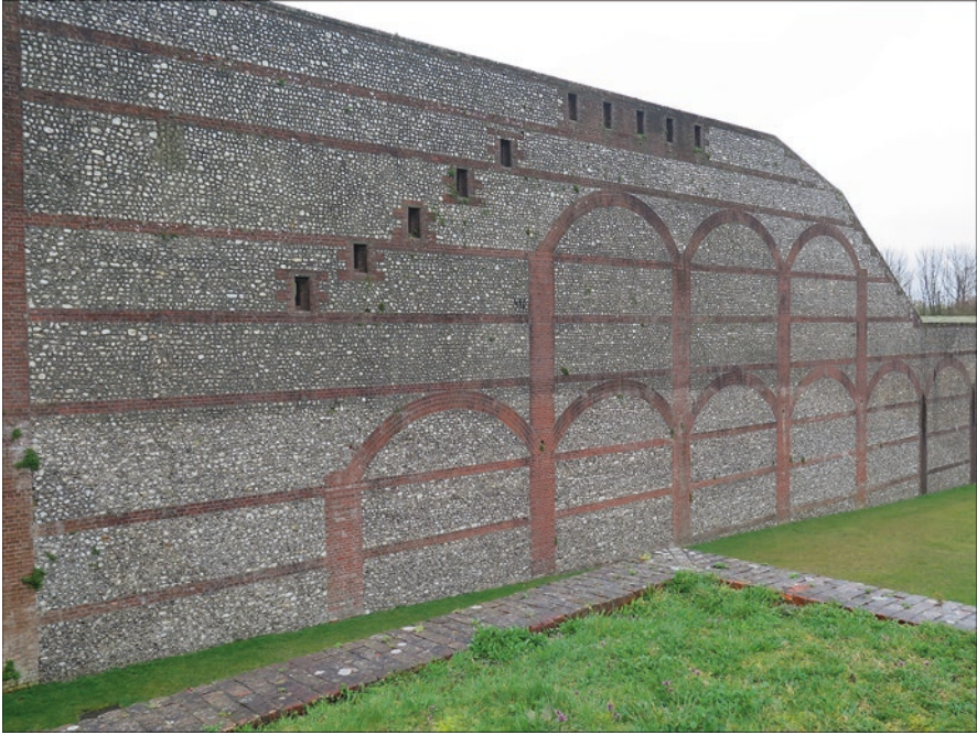
Fig. 3.15 The flint and brick inner wall of the ditch surrounding Fort Nelson
