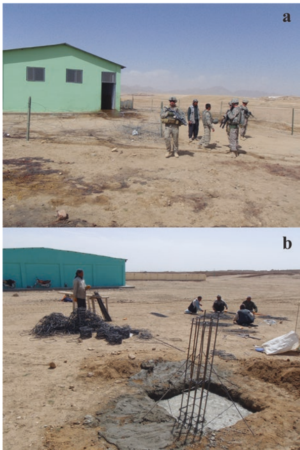
Fig. 14.4 Ground photographs of the Ghazni Agricultural Complex in March 2009. (a) This photo looks westerly at the recently built slaughterhouse (red arrow on Fig. 14.3); note the blood-stained ground (especially front left). (b) This photo is easterly facing showing the new foundation emplacement for the sales barn (yellow arrow on Fig. 14.3)
