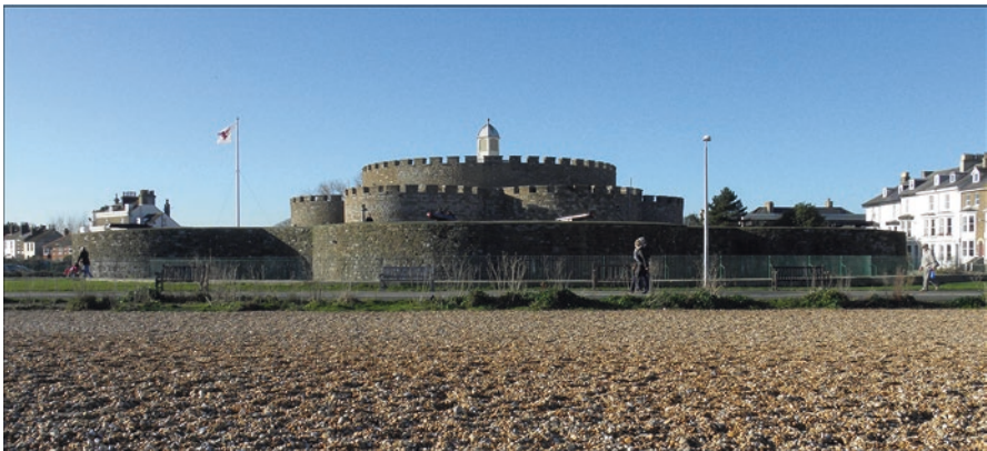
Fig. 3.3 Deal Castle, Kent, a typical low-profile, thick-walled Henrician fort viewed from the beach
