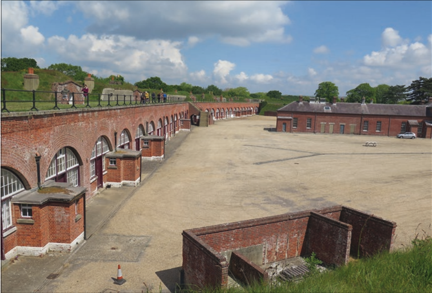
Fig. 3.11 Parade ground at Fort Brockhurst, Gosport, Hampshire, with casemated barracks on the left below the ramparts
