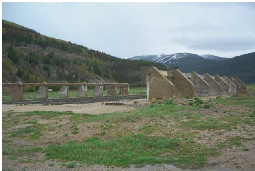
Fig. 11.3 Remaining structures (field house) at Camp Hale (Doe 2011)
