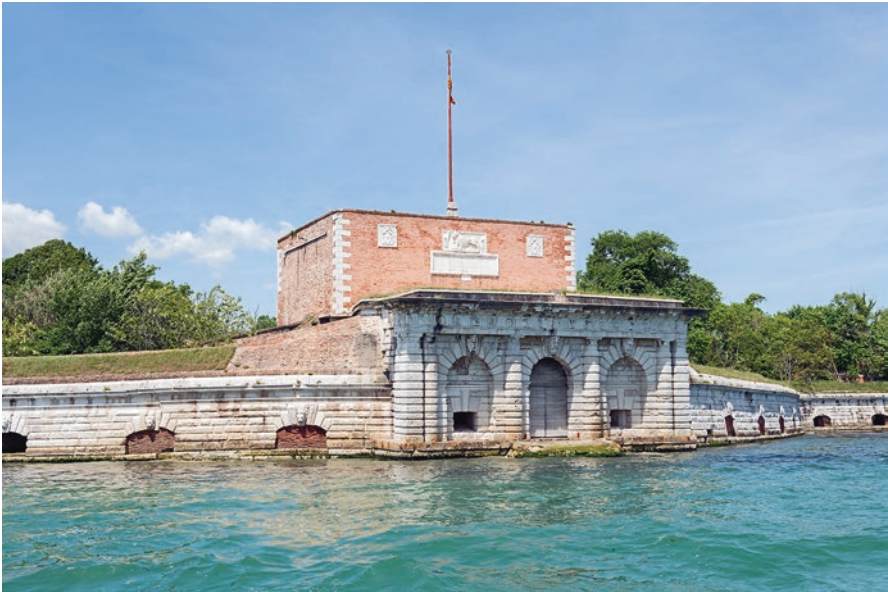
Fig. 1.2 The Fort of Sant’ Andrea in the Venetian Lagoon. The fort protected the entrance to the lagoon from the Lido inlet. It was built by Michele Sanmicheli between 1545 and 1550 and completed in 1571 by Francesco Malacrida on the remains of previous defensive works and is a part of the lagoon defensive system (photo by Didier Descouens; Wikimedia Commons, CC BY-SA 4.0)
