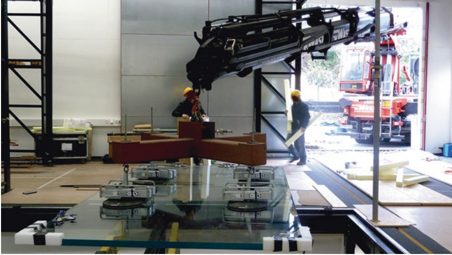
Fig. 9.13 Complex installation of the glass plates for the floor rear projection of the aixCAVE. (© TW Kuhlen, G Matthys. All rights reserved)
