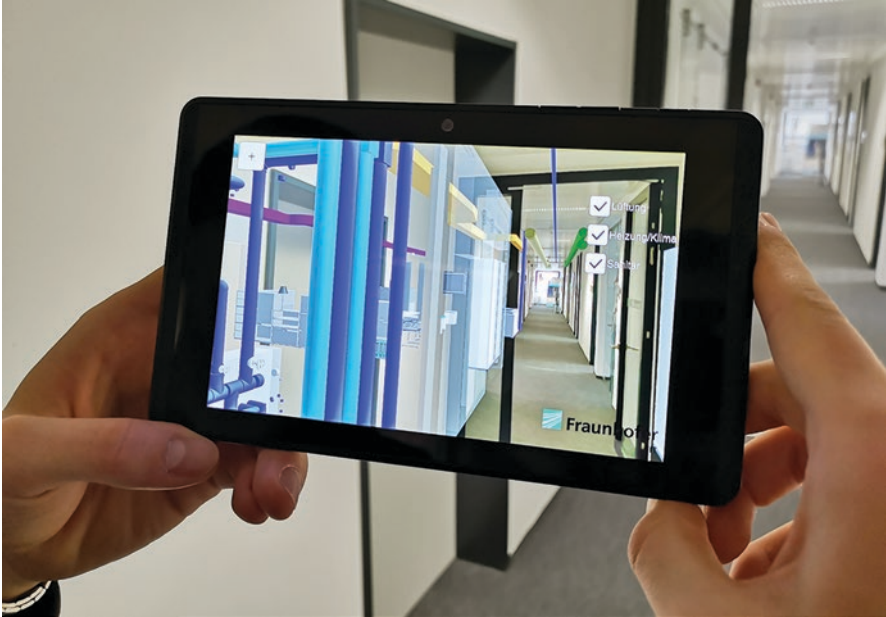
Fig. 8.24 Pipes and cables behind a cover and in the wall are made visible using AR for X-ray vision. (© Leif Oppermann, Fraunhofer FIT 2018. All rights reserved)
