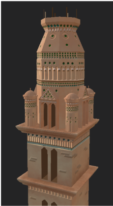
(a) Bell Tower
