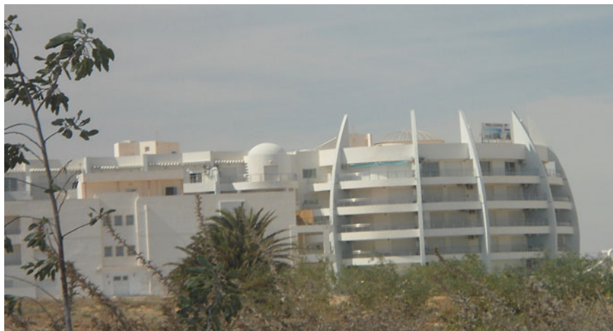
Fig. 5 The para-hotel project “Hergla Diamant.” Source M. Hellal, November 2019
