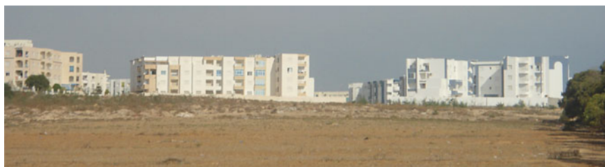
Fig. 4 The AFH “Corniche-Hergla” Housing Project. Source Photographed by M. Hellal, November 2019
