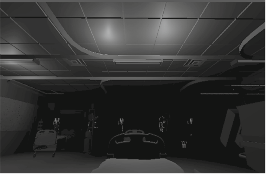
Fig. 7. Before the appearance of insects on the ceiling.
