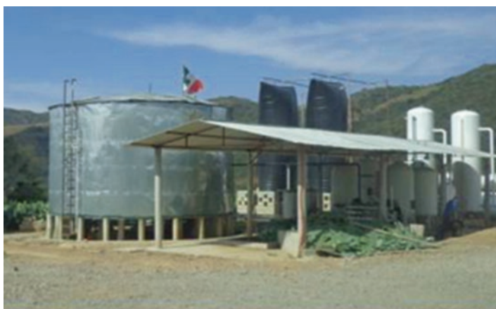
Fig. 43.2 Biogas generating plant from O. ficus indica
