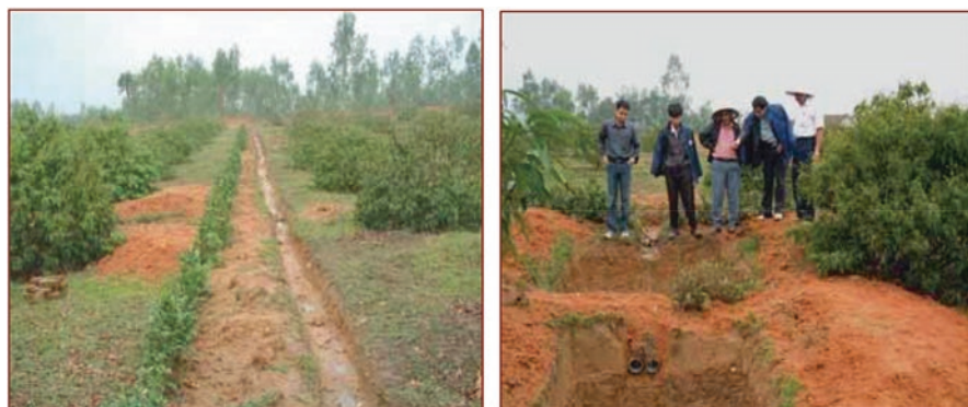
Fig. 13.17 Contour trenches (left) and groundwater recharging structures (right) in Vietnam. (Source: Authors)
