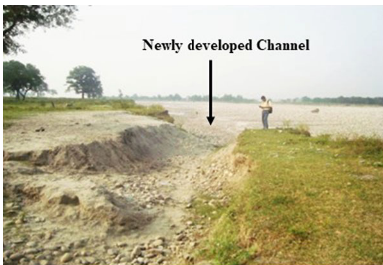
Fig. 8.16 A newly developed channel along the left bank, at Haridwar, after the flood hazard in Ganga River, Nildhara area. (Source: Field survey, October, 2013)
