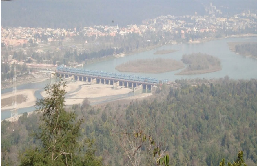
Fig. 8.17 Bhimgoda barrage at Haridwar to divert Ganga water into the upper Ganga canal, influencing excessive channel sedimentation and interruption in channel equilibrium. (Source: field survey, February, 2010)
