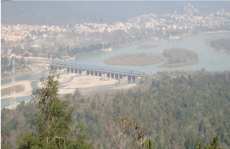
Fig. 8.17 Bhimgoda barrage at Haridwar to divert Ganga water into the upper Ganga canal, influencing excessive channel sedimentation and interruption in channel equilibrium. (Source: field survey, February, 2010)
