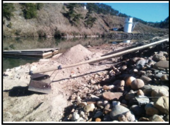
Fig. 11.4 Bar skimming method of sand mining (25°27'47"N to 91°49'40"E)
