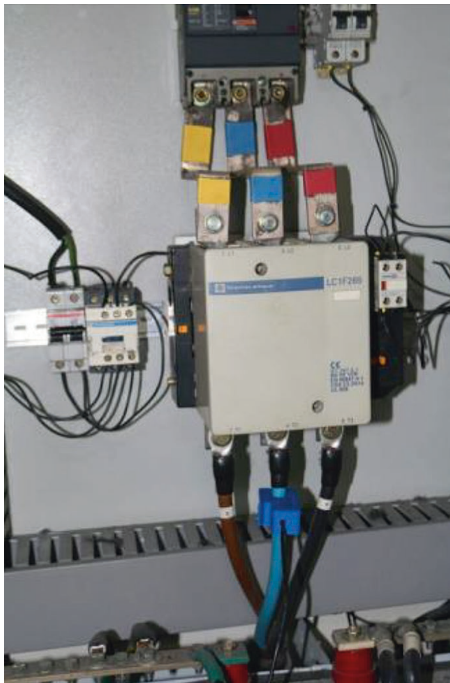
Fig. 7 Installing the current sensor
