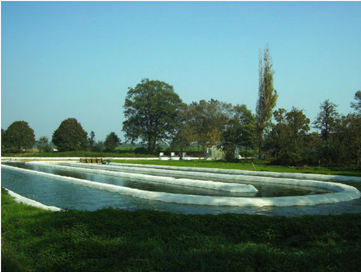
Fig. 3 Microalgal open system: high rate algal pond
