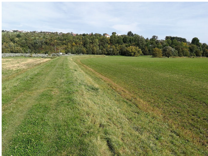
Fig. 4 Flood dike delimiting the polder area (on the right side), as an inundation area of the Dřevnice River on the outskirts of Zlín City, Czech Republic
