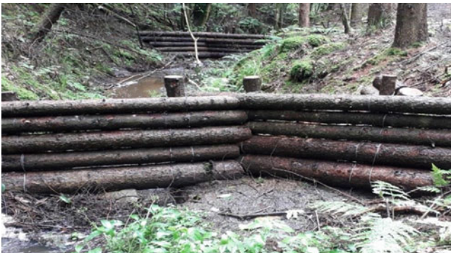
Fig. 9 Leaky barriers structure applied in the torrential river, after Hankin et al. [19]
