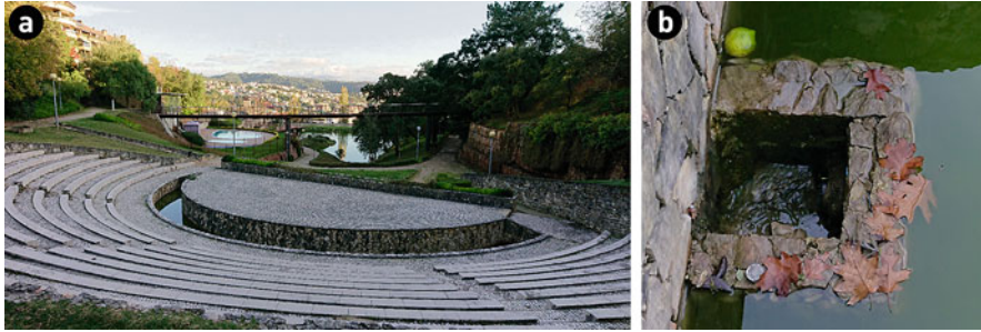
Fig. 5 View of the Amphitheatre in the foreground, with a small water retention volume (a), and the reduced outlet connecting to the settling ponds (b)
