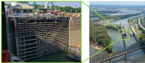
Fig 1a: Locks and miter gate
