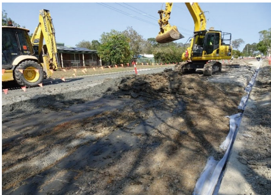
Fig. 10 Photograph of high-plasticity subgrade site tested with IC technology
