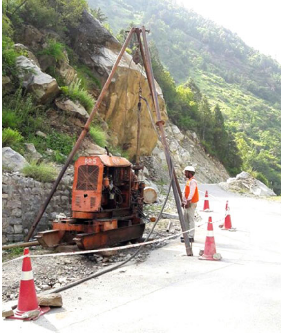
Fig. 4 Borehole drilling in progress
