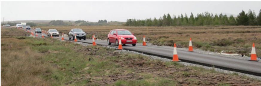
Fig. 10 N56 floating cycleway during use as a temporary diversion route
