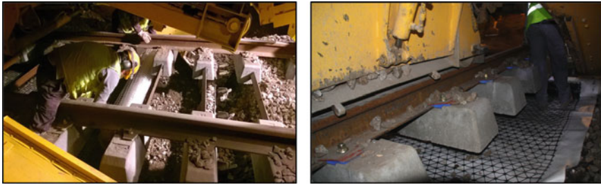
Fig. 3 Application of geotextile and geogrid [14]
