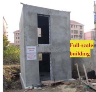
(f) The photo of the two-story building.
