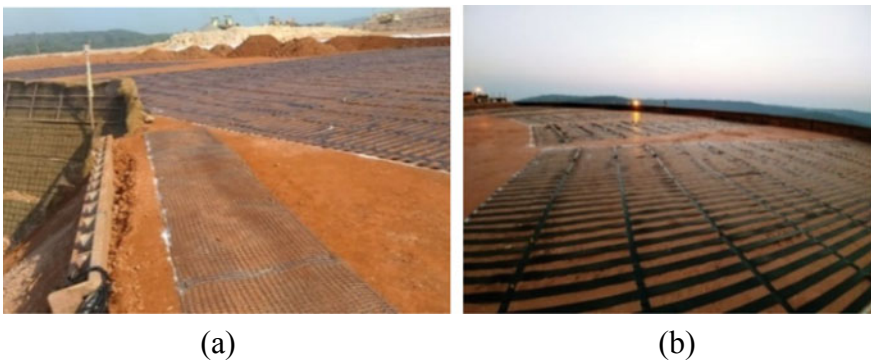
Fig. 12 Geogrid arrangement at: a convex face; b concave face
