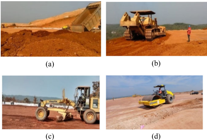
Fig. 10 Construction activities: a dumping; b dozing; c grading; d compaction
