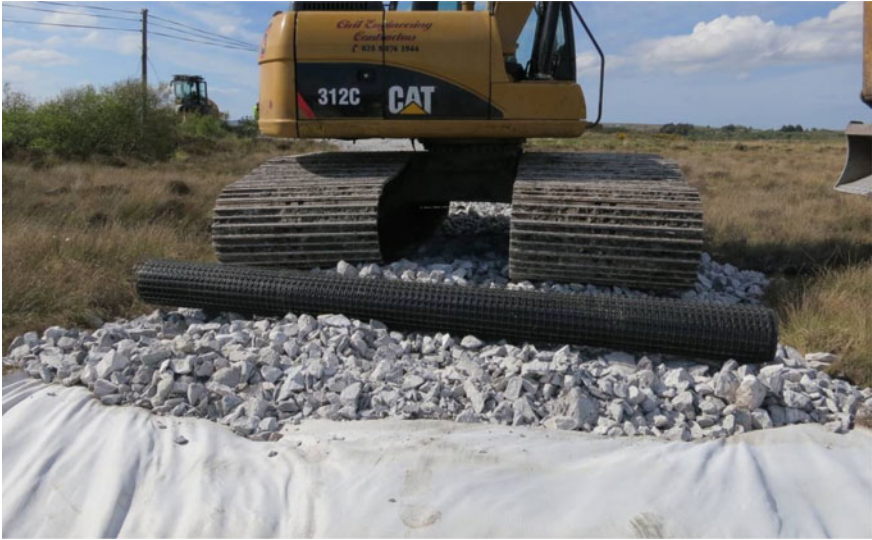
Fig. 9 N56 floating cycleway during construction
