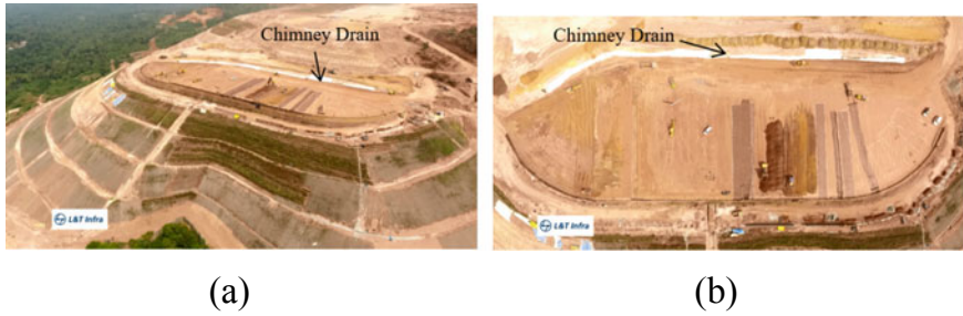
Fig. 13 Aerial view of chimney drain alignment in 5th tier
