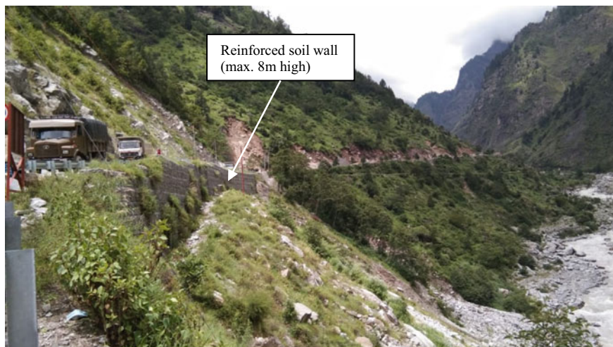
Fig. 20 Photograph showing reinforced soil wall constructed at site for road retention
