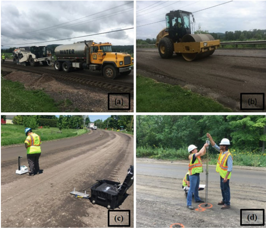
Fig. 1 Photographs of a reclaiming, b compacting, c NGD, and d DCP test
