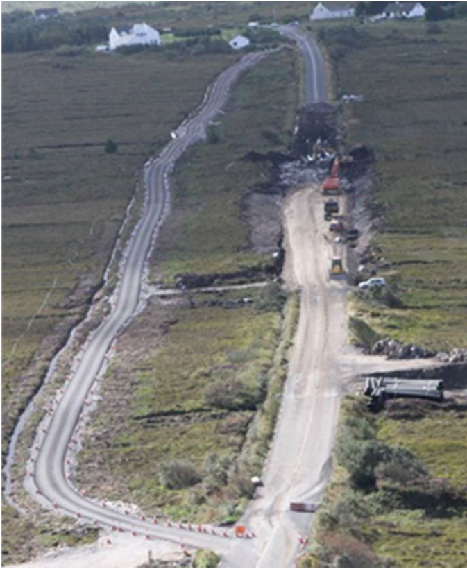
Fig. 8 N56 floating cycleway during construction
