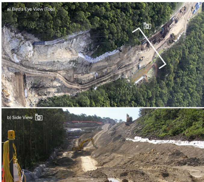
Fig. 2 Aerial view of site (a) and side view looking west (b)
