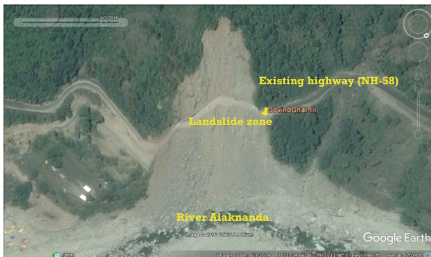
Fig. 2 Satellite image in 2014 shows major landslide above and below the highway
