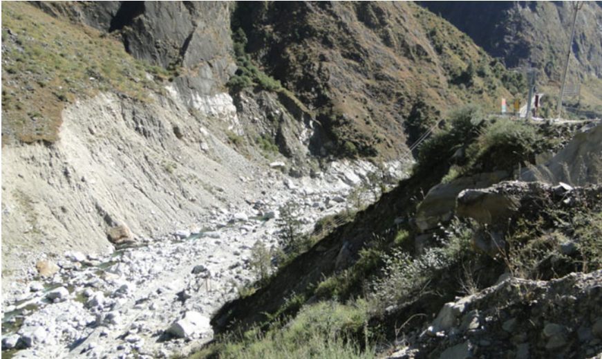
Fig. 10 Toe erosion on valley side
