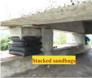
(c) The installed stacked sandbags.
