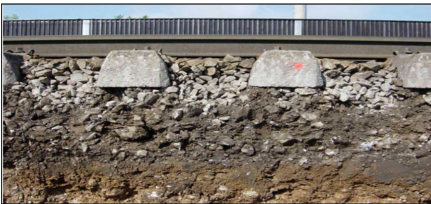
Fig. 2 Cross-section of the ballasted rail track [14]
