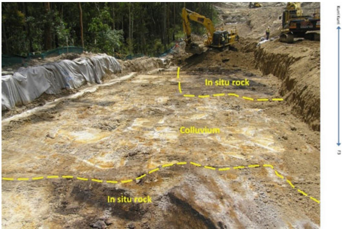
Fig. 7 RSW foundation exposing different materials: in situ rock and compacted colluvium
