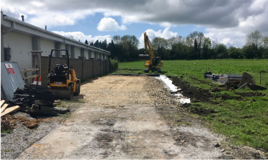
Fig. 11 Temporary access road at retail development site, Birr, County Offaly
