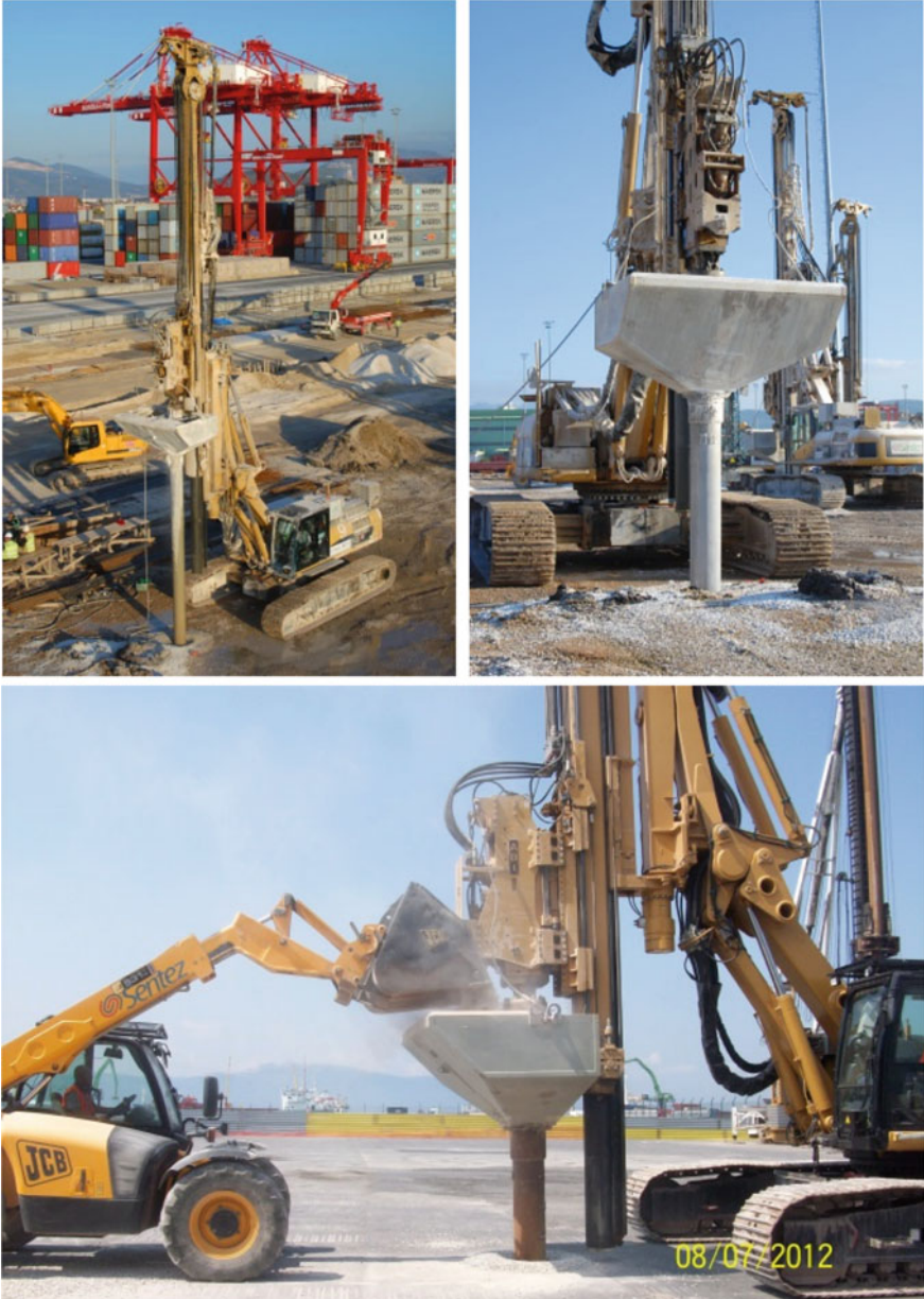
Fig. 2 Rammed aggregate pier® installation
