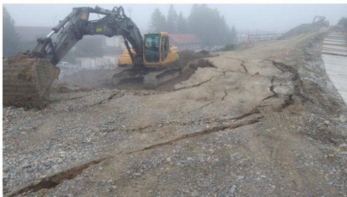
Fig. 12 Slope adjustment without free cut
