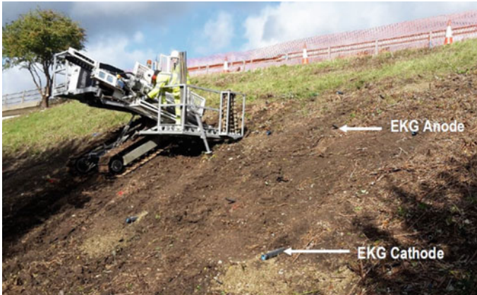
Fig. 3 P45 Slope climbing drill rig installing electrodes: A419 Rat Trap, 2014 [4]
