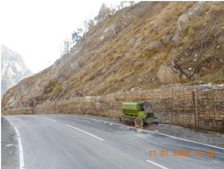
Fig. 19 Photograph showing the hill side rehabilitative measures 3-m high nailed gabion wall for toe stabilization and secured drapery system to secure large boulders adopted at site
