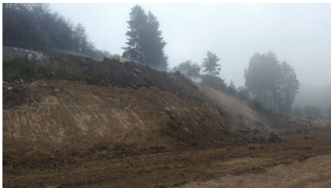
Fig. 11 Slope adjustment without free cut
