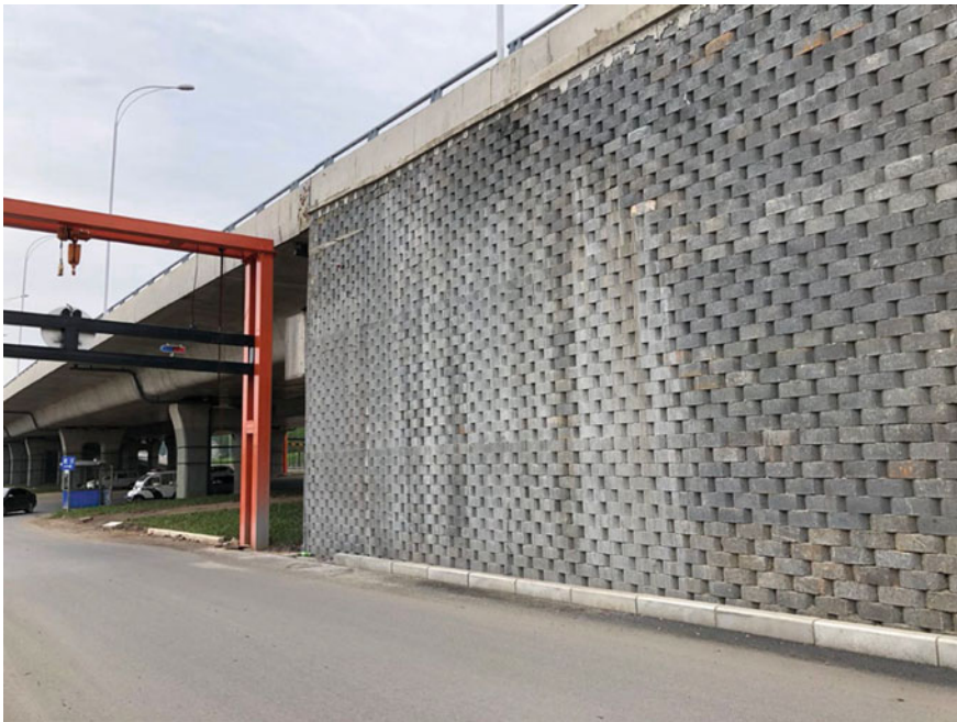
Fig. 1 Overview of the GRS bridge approach during the service period
