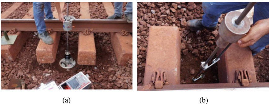
Fig. 2 Characterization aspects at km 538 + 250 m with (a) LWD and (b) DCP
