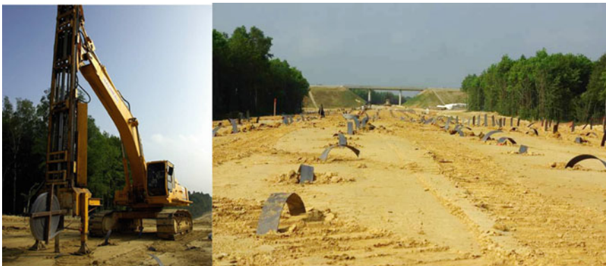
Fig. 3 Installation of the vertical wick drains
