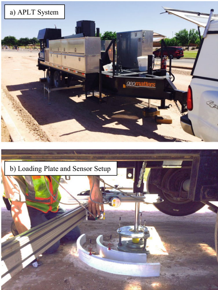
Fig. 3 Automated plate load testing (APLT)
