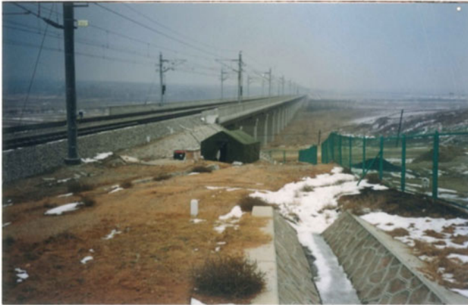
Fig. 1 Overview of the bridge-subgrade transition zone (DK 43+578)
