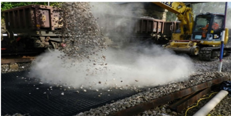
Fig. 5 Installation of geogrid + APG at Bradley Junction
