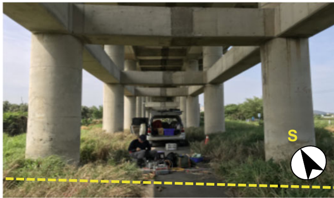
Fig. 9 Inspection line of electrical resistivity tomography along pile bents
