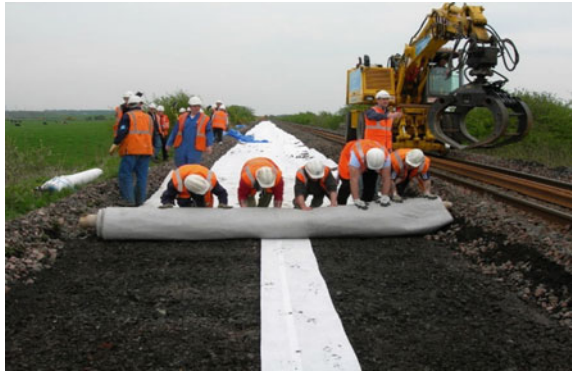
Fig. 1 Installation of a 15 m roll of geosand
