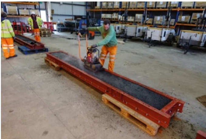
Fig. 1 Asphalt tray being loaded with asphalt and compacted
