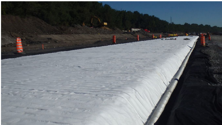
Fig. 11 Installation of the draintube drainage geocomposite
