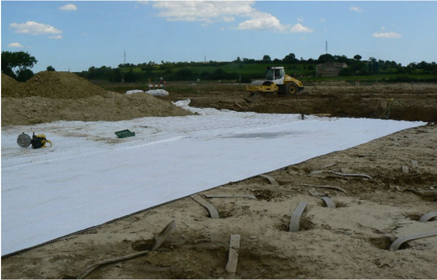
Fig. 4 Drainage geocomposite installation
