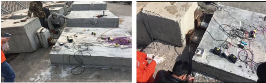
Fig. 4 Counter force wall and jack site layout diagram
