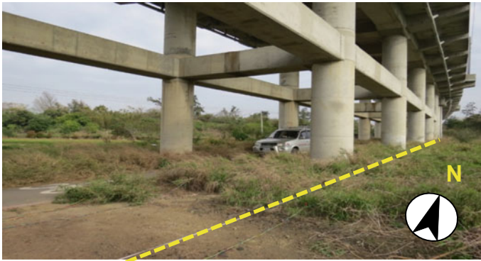
Fig. 6 Inspection line of electrical resistivity tomography along the rail bridge
