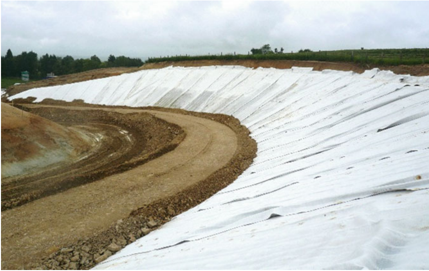
Fig. 6 Drainage mask construction with drainage geocomposite
