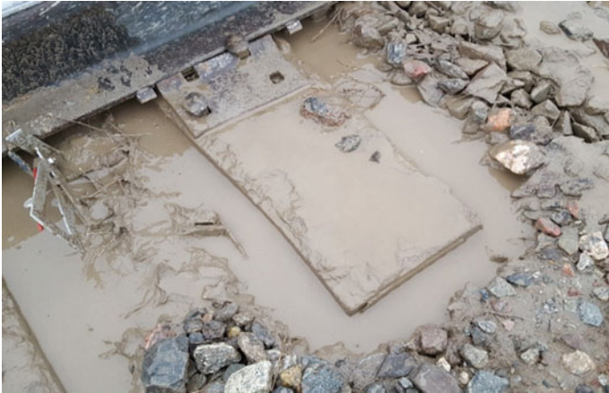
Fig. 4 Photograph of mud pumping with standing water
