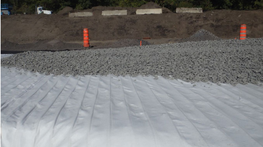
Fig. 12 Backfilling of the product with ballast
