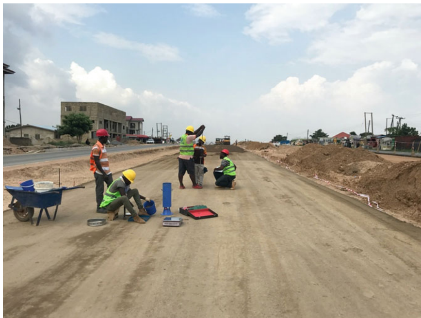
Fig. 5 Quality control testing on permanent works
