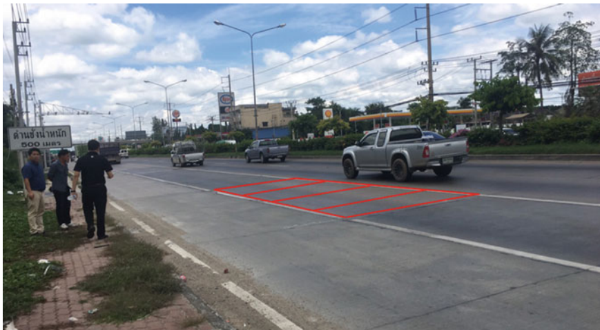
Fig. 2 A field instrumented rigid pavement section
