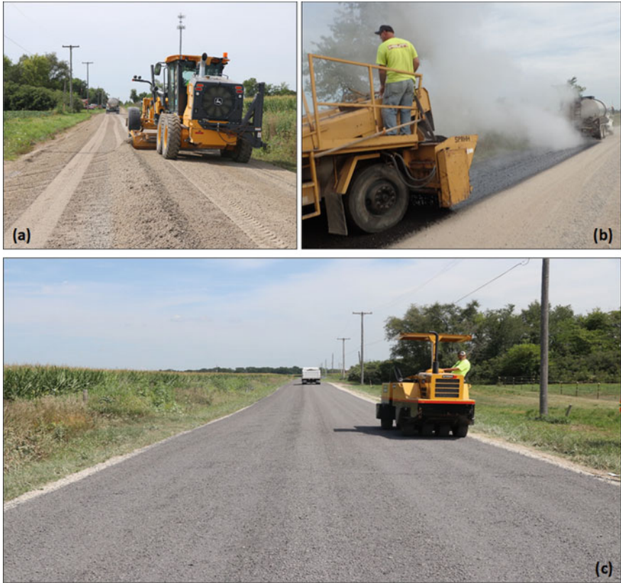
Fig. 2 Otta seal construction sequence in Louisa County, IA using slag
