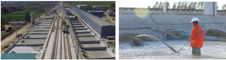
Fig. 11 Site construction picture of foamed lightweight soil subgrade widening
