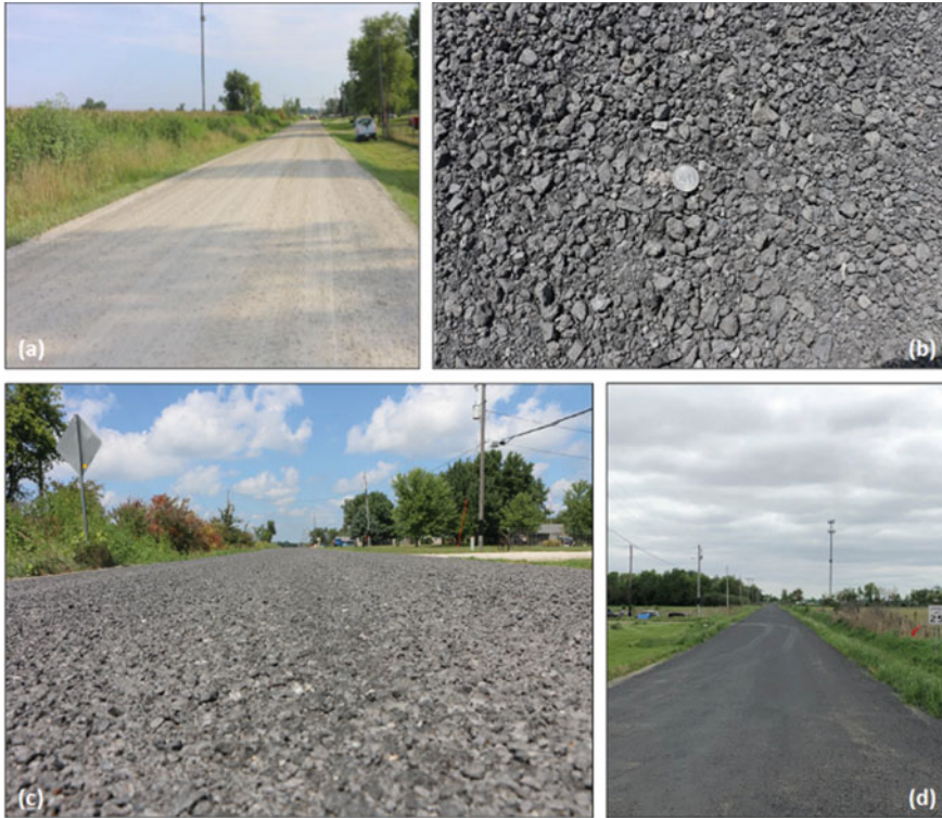
Fig. 4 Appearance of the slag Otta seal on 142nd Ave. in Louisa County, IA a before construction, b immediately after construction, c one month after construction, and d eight months after construction
