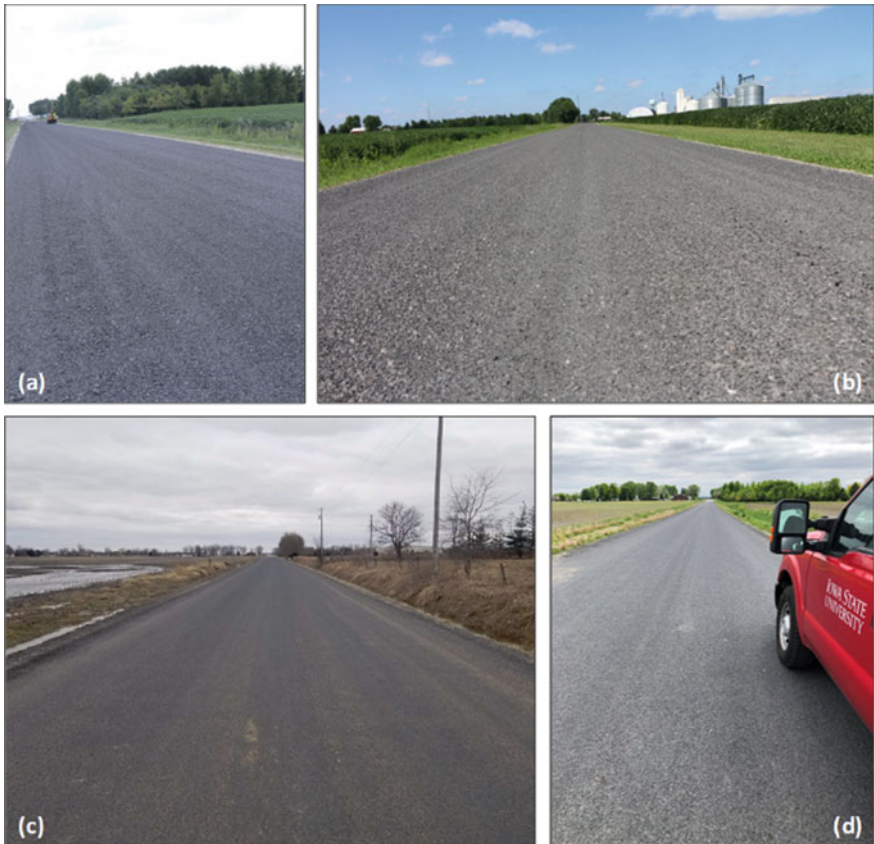
Fig. 3 Appearance of the slag Otta seal on K Ave. in Louisa County, IA a immediately after construction, b one month after construction, c eight months after construction, and d ten months after construction
