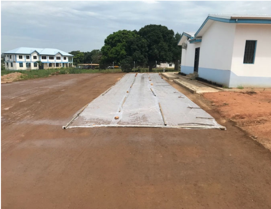
Fig. 3 Curing of laid CSSB in the yard
