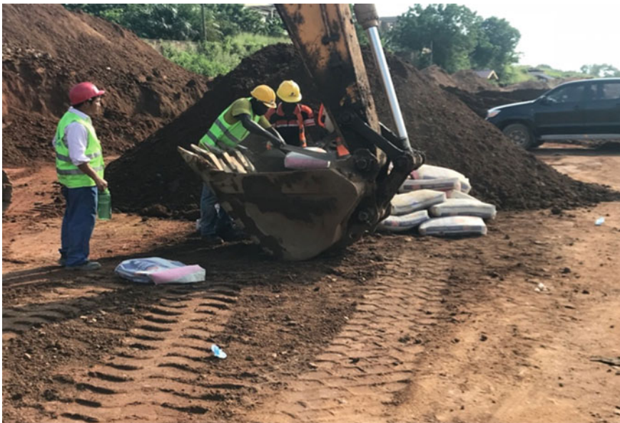
Fig. 2 Batching of lateritic soil and cement in the yard
