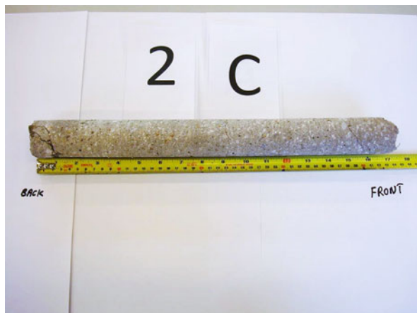
Fig. 11.32 Core taken from fire-damaged area
