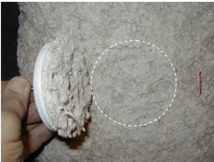
Fig. 5.13 SFRM cohesion failure (during a pull test) [25]
