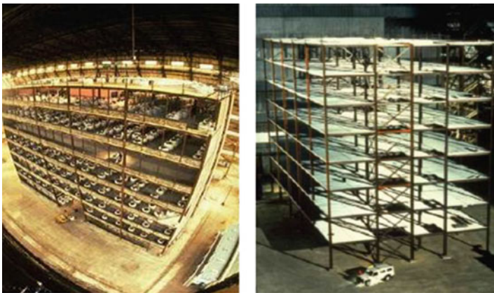
Fig. 7.5 Cardington test building [20]
