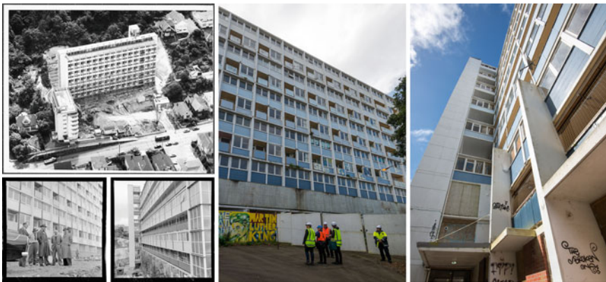
Fig. 13.2 Photographs of the Gordon Wilson Flats from the 1950s (left), and photographs of the building currently (right)
