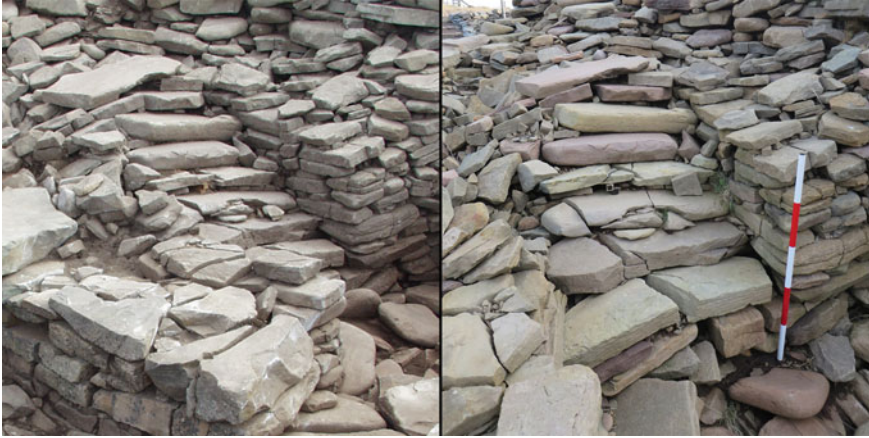
Fig. 14.20 Left, top-down view photograph of the north stair taken in 2003. Right, side view the same stair in 2015. Note how the wooden pinnings supporting the fourth step are in different positions, suggesting stone movement, small loose stones are in different positions. The angle of the photographs is different, as is the perspective of the shots, which makes like for like visual comparison of the steps difficult through studying only the original photographs, although there are some certain differences in loose stones being in different locations (V.E. Turner, Shetland Amenity Trust)
