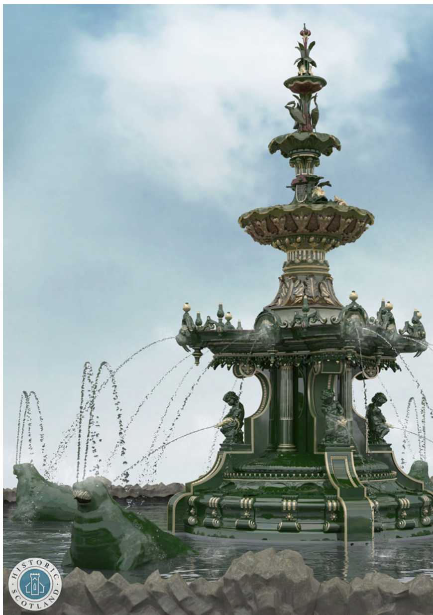
Fig. 16.6 Visualisation of the original paint scheme based on scientific analysis of original paint scheme and 3D model derived from laser scan point cloud
