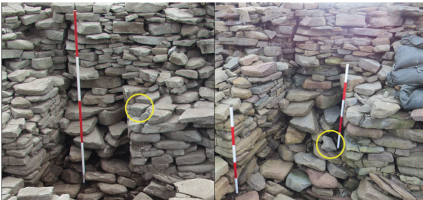
Fig. 14.16 Left, top-down view entrance passage in 2003. Right, side view entrance passage in 2015. Note how a stone from the wall top on the western side of the passage has fallen into the passage itself and is located beside the range pole (circled in yellow) (V.E. Turner, Shetland Amenity Trust)
