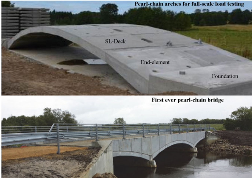
Fig. 3 Top: SL-Deck elements and end-elements post-tensioned together in an arch shape. Used for full-scale load testing. Bottom: first ever constructed bridge based on arches using the pearl-chain method
