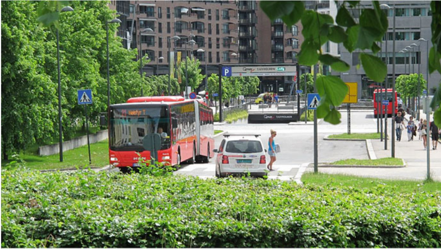
Fig. 11 Pedestrian crossings on speed platforms (Oslo, Norway)
