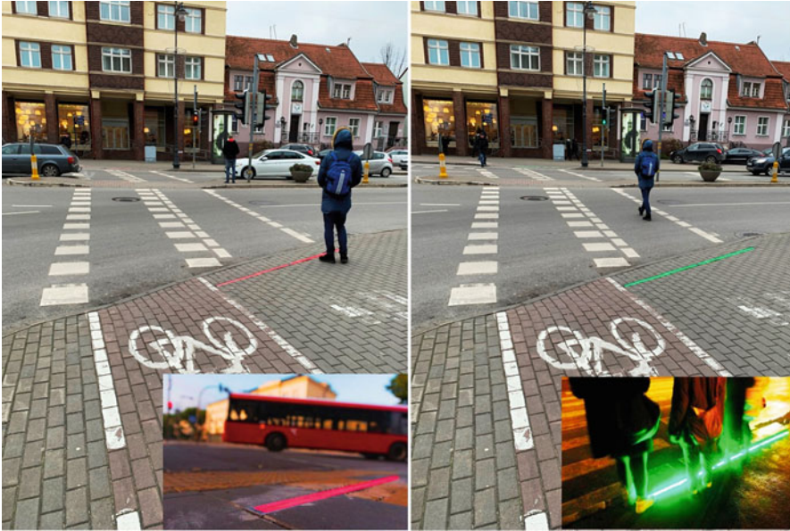
Fig. 8 Pavement LED stoplight strips are mounted to duplicate traffic lights and draw the attention of pedestrians using phones
