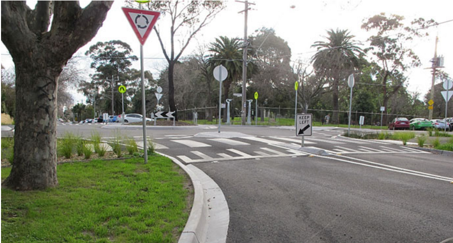
Fig. 13 Urban local street roundabout with elevated pedestrian crossings (Melbourne, Australia)
