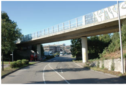
a. Overview of the bridge.
