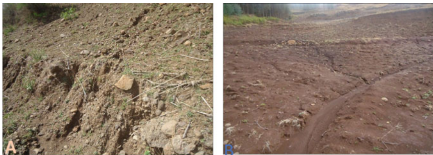
Fig. 17.3 Rill erosion formed in poorly constructed soil bund in Dibakuhan watershed (a). Earth crusting, smoothing of cultivated land and rills formed in Andit Tid watershed (b)
