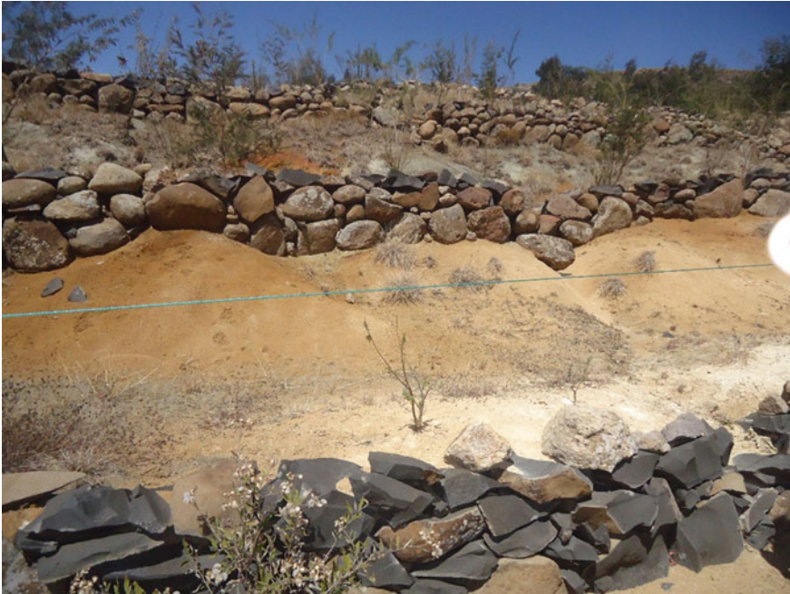
Fig. 17.12 Newly constructed hill side terrace in Nekubish watershed
