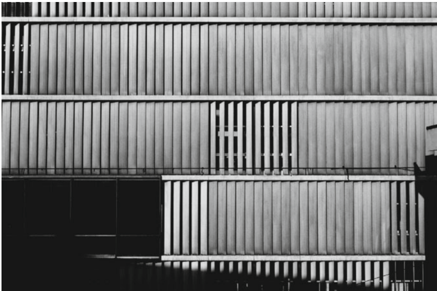
Fig. 13 Detail of louvers sunshades on the main façade. The different approach used in the boardroom on the second floor is marked by the brise-soleil absence (source Associazione Archivio Storico Olivetti, Ivrea—Italy, Fondo Fototeca/Foto Miscellanea Olivetti)
