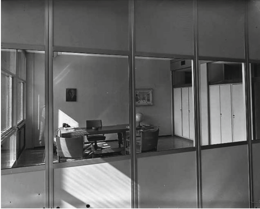
Fig. 20 The “Anacustic” removable partition walls. In the background, one of the offices and the succession between doors and closets ( source Associazione Archivio Storico Olivetti, Ivrea—Italy, Faldone 26)
