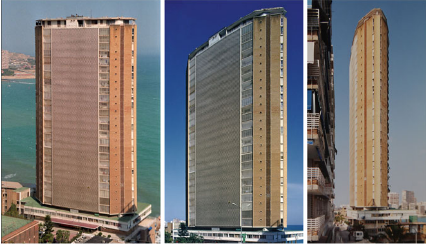
Fig. 13 Three views of the rear façade (facing the road) of the Vistamar tower with the large lattice (Authors, ca. 1996)
