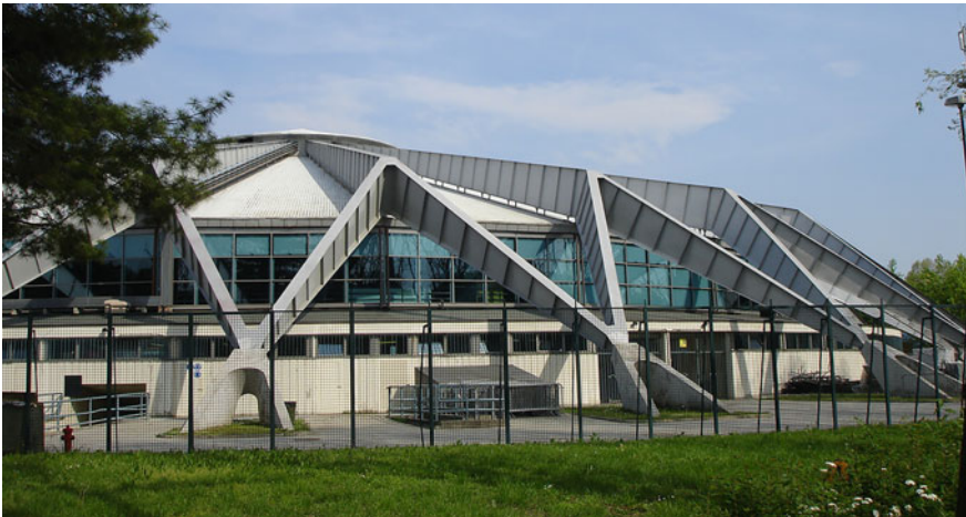
Fig. 4 The Palazzo dello sport in Turin. A. Vitellozzi. 1960–61. External view (photo by the autor)
