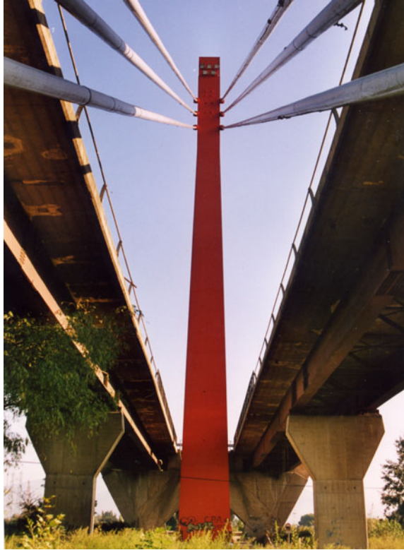
Fig. 17 The cable-stayed bridge over the Arno river. A. Montemagni, P. Sica, F. de Miranda. 1969–1978. Executive design (Archive “Studio de Miranda Associati”)
