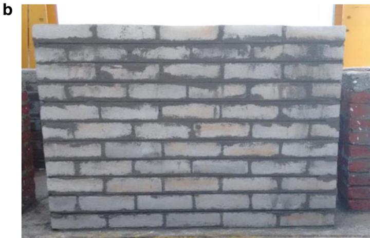
**Fig. 17.28** a Schematic representation of typical geopolymer solid block wallette. b Stretcher bonded solid block wallette kept for curing
