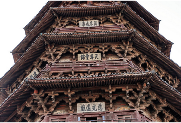
Fig. 5. Clusters of brackets under the eaves of a wood pagoda in Ying 应 county, North China. Source: author.
