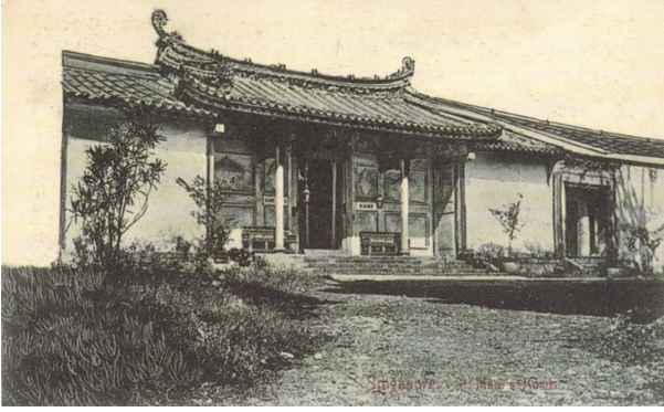
Fig. 8. Postcard of St. Mary's Home (c. 1920) shows that its main entrance's front elevation had no window opening to the exterior (public domain).
