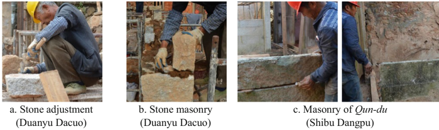
Fig. 12. Composition of stone masonry.
