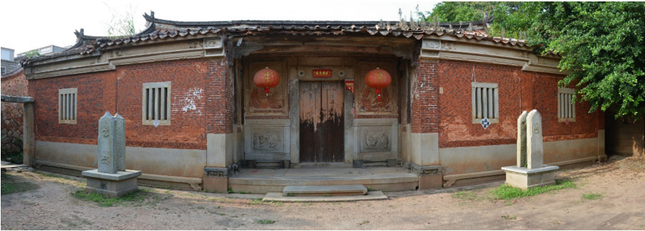
Fig. 7. Photo of a typical Jing-mian wall (Kaitai Jinshidi).
