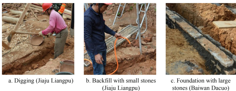
Fig. 11. Composition of the masonry at the base of the wall.
