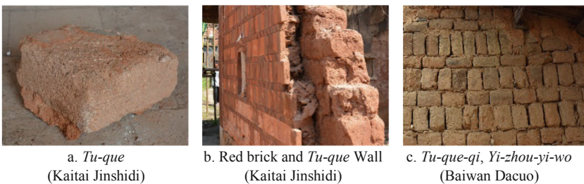
Fig. 5. Examples of the use of Tu-que in traditional architecture.
