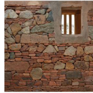
b. Interior wall (Xiuhualou)
