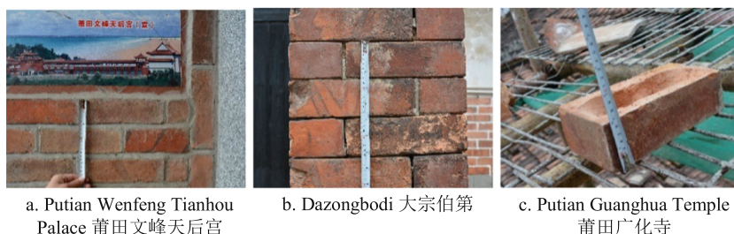
Fig. 19. Types of red brick used in Putian.
