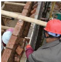
a. Masonry of Feng-zhuan-bi
