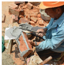
b. Plaster placed at the edges of bricks
