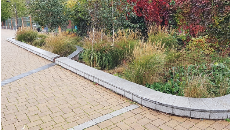
Fig. 9.5 An example of a well-adopted Sustainable Drainage System (SuDS). Consideration for the SuDS stewardship means that it is well-managed and considered to be a valuable asset by the local community
