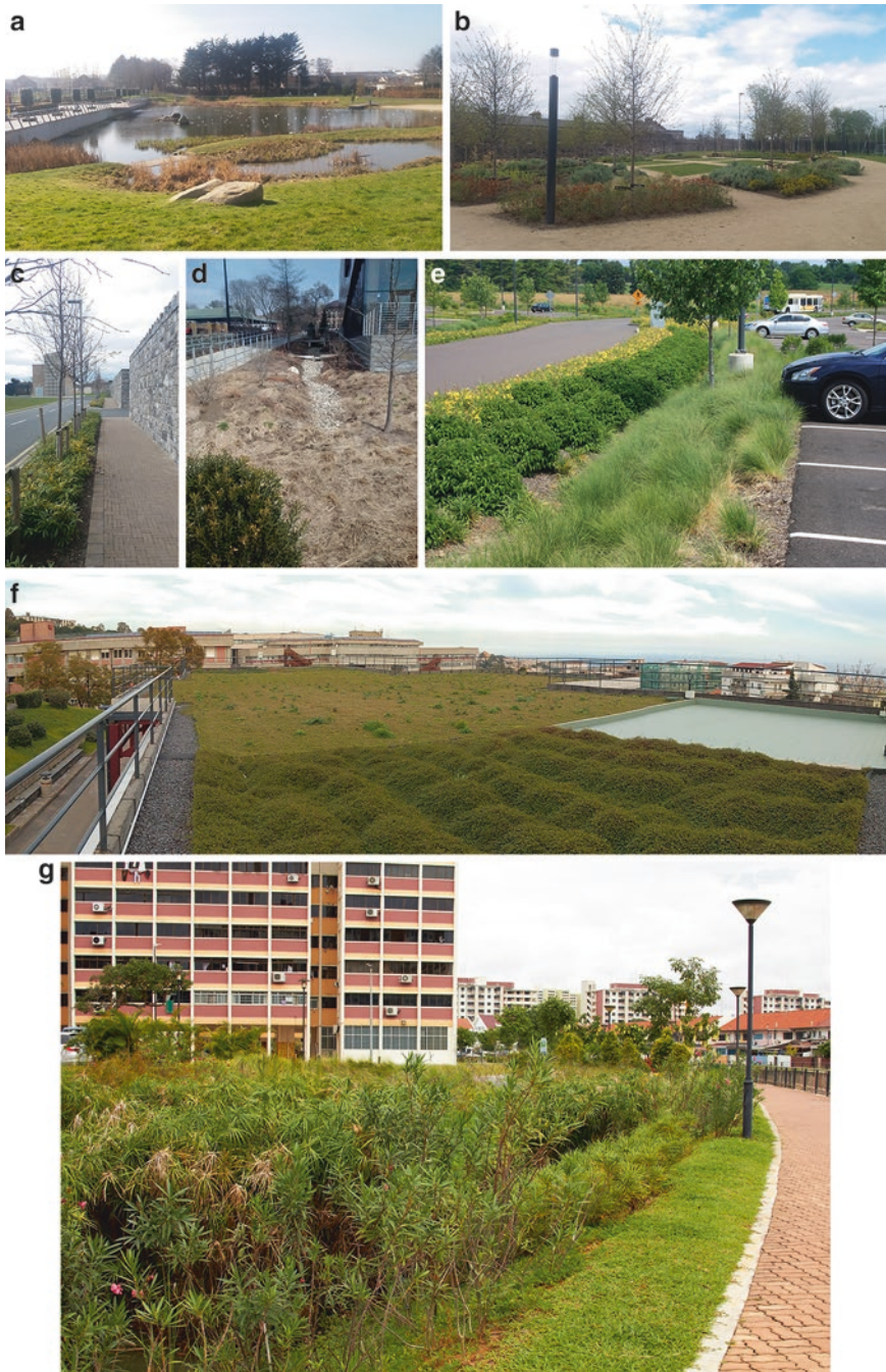
Fig. 16.1 Examples of Sustainable Urban Drainage Systems. (a) Detention basin in Dun Loghaire (Ireland); (b) Permeable pavements in Dublin (Ireland); (c) Filter drains/strips in Dublin (Ireland); (d) Swale in Amherst (USA); (e) Infiltration trenches in Pennsylvania; (f) Green roof in Catania (Italy); (g) Rain garden in Singapore. (a–d and f) Photo credit: the authors; (e) Photo credit: Montgomery County, under Creative Commons License (CC BY-SA 2.0); (g) Photo credit: Roger Soh, under Creative Commons License (CC BY-SA 2.0)
