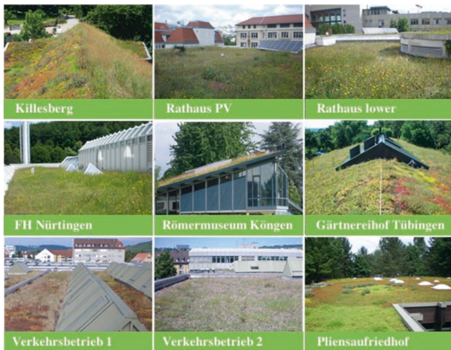
Fig. 10.4 The nine EGRs surveyed were all multi-layered systems with under 10 cm substrate depth
