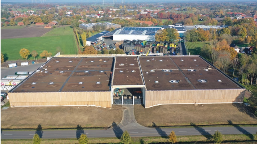
Fig. 6.3 Construction of a 1 ha-wide green roof with different substrate depths (8–15 cm) and biodiversity elements in Wagenfeld, north-western Germany, in autumn 2019. Dry grassland species were sown on shallow substrates and mesophytic species on areas with higher substrate depth. (Photo credit: Hermann Tegeler, provided by Friedrich Lütvogt GmbH & Co. KG)
