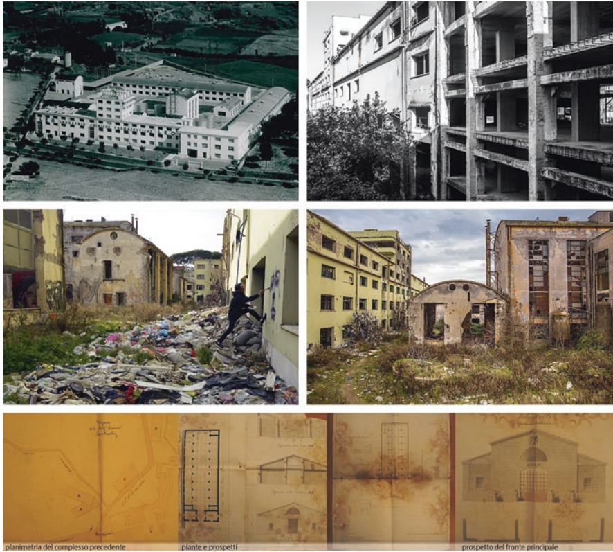
Fig. 22.1 Historical photographs and drawings of the case studies. Above: Leo Factory in 1950 (left) and 1959 (right)
