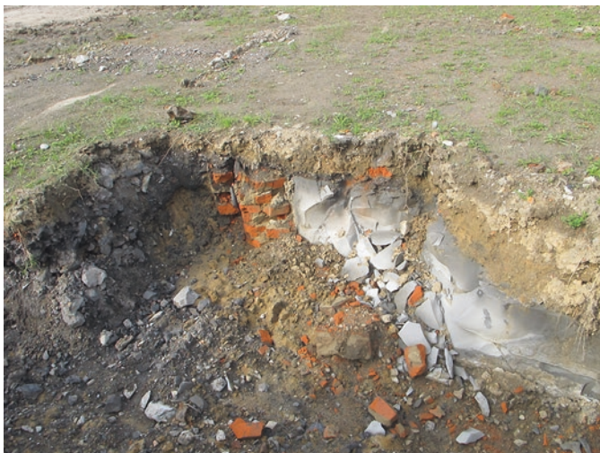
Fig. 11.3 The quality and the continuity of urban soils is seriously compromised by the presence of pre-existing structures and services. This hinders the healthy development of most of the plants growing on such substrates
