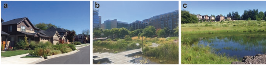
Fig. 26.2 Constructed wetlands come in different sizes and degrees of naturalness. (a) Small, concrete street-side rain gardens treat stormwater from the adjacent road. (b) Medium-sized wetland parks treat water from apartment buildings in a dense urban core. (c) Large constructed wetlands treat stormwater from an entire suburban neighbourhood
