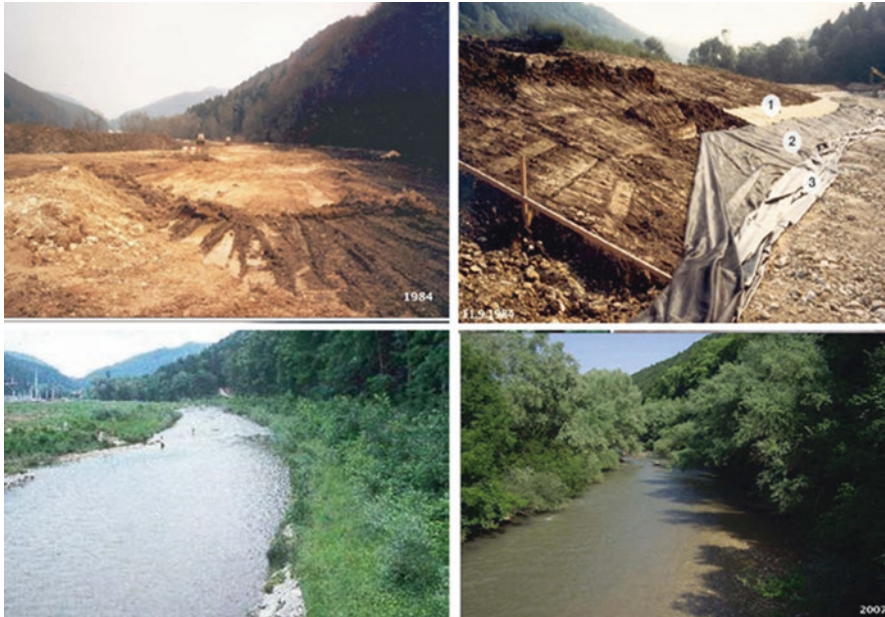
Fig. 17.1 Evolution of the work carried out on Byrse River: comparison of images from 1984 to 2007. (Photo credit: B. Lachat)
