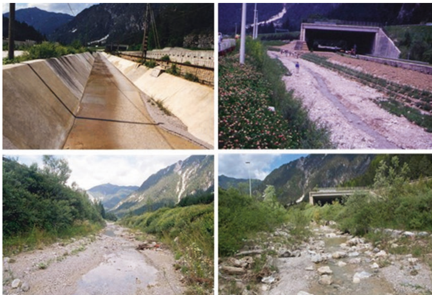
Fig. 17.2 Evolution of the work carried out on Fella River (Italy): comparison of images from 1994 to 2016. (Photo credit: G. Sauli)
