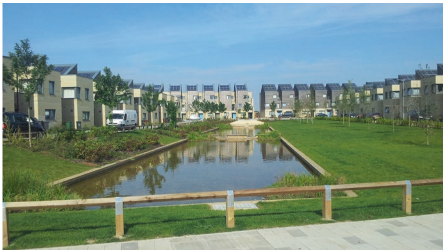
Fig. 9.4 An example of nature-based solutions within the public realm of the Barking Riverside development. The stewardship of this amenity, biodiversity, and stormwater management area will be taken over by the Community Interest Company. (Photo credit: Stuart Connop)
