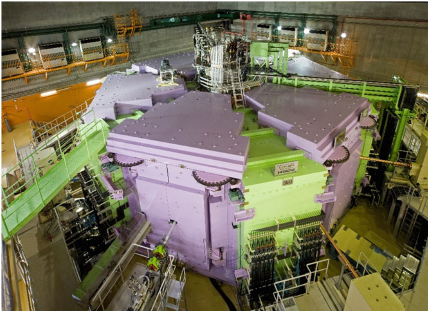
Fig. 10.22 SRC after assembly in the vault. The control liquid helium Dewar is seen on the top in the centre of the cyclotron (Courtesy Hiroyoshi Sakurai and with permission from RIKEN Nishina Centre and iTHEMS Promotion Office) https://ribf.riken.jp/RIBF-TAC05/1_Overview.pdf
