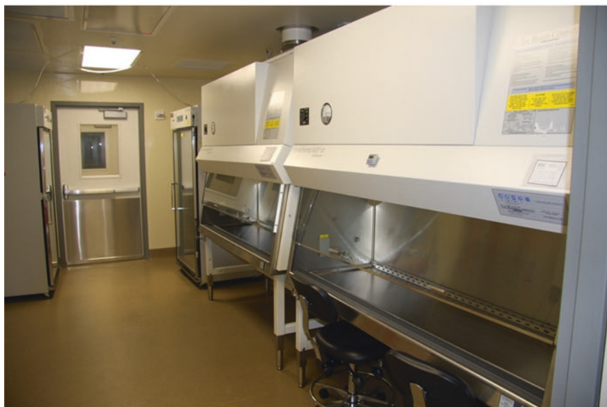
Fig. 3 Pre-production area (top) and production suite (a) Pre-production area. The four doors on the left-hand side lead into the production suites. The doorway to the right is the entry to the storage room. The door at the far end leads from the materials entry anteroom into the pre-production area. (b) One of the four production suites containing two biosafety cabinets
