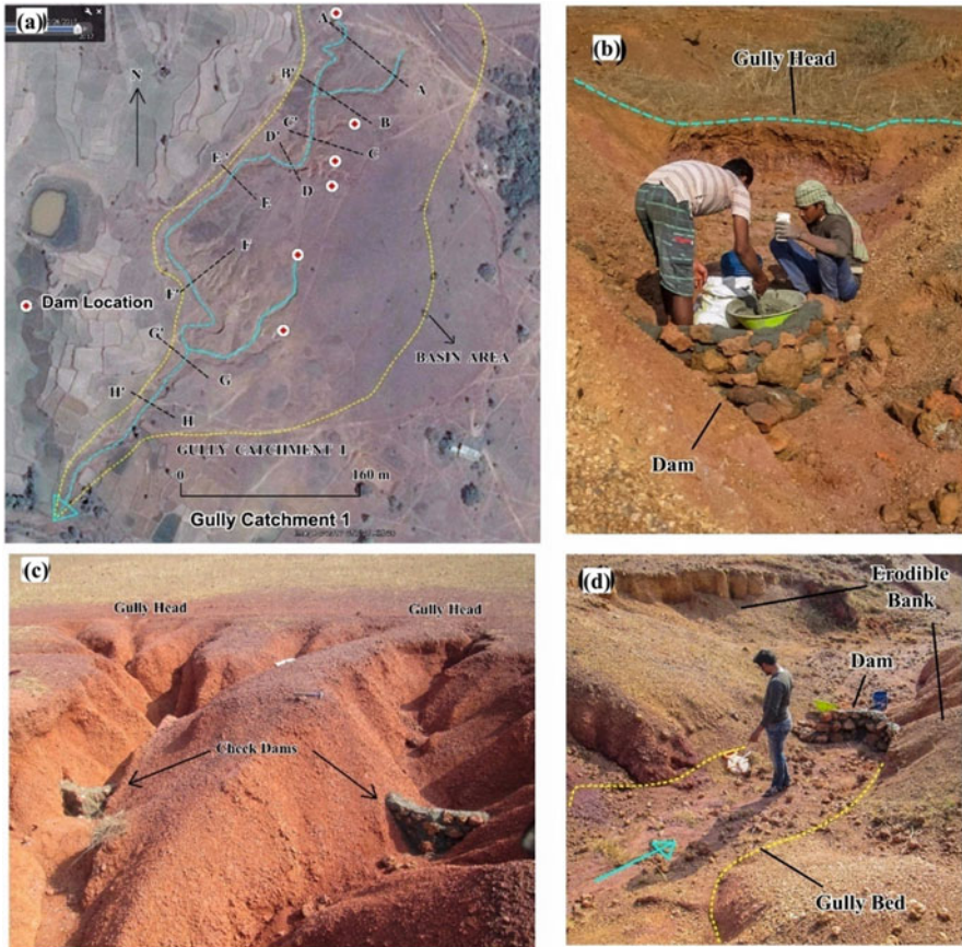
Fig. 7.6 (a) Sample dam locations at gully headcuts in catchment 1, (b) development of temporary dam to trap sediments, (c) final structure of small dams below gully headcuts and (d) measuring the morphological parameters above dam
