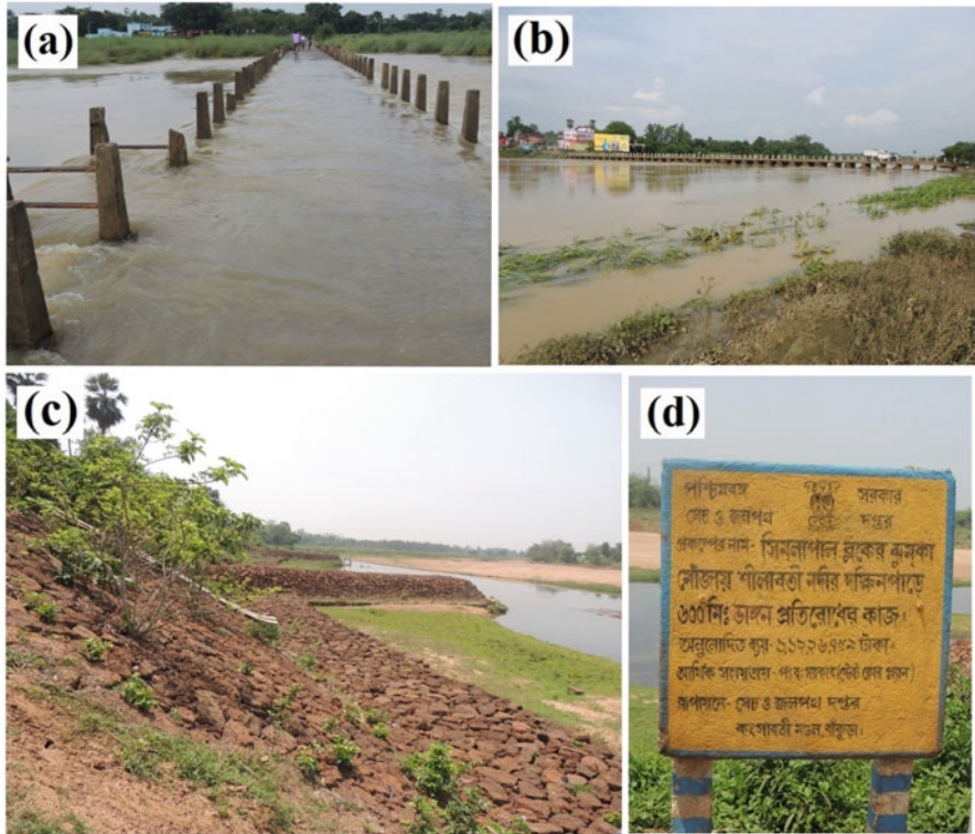
Fig. 6.17 (a) Flood water spilling over the road near Bhelaidiha, Bankura on 25th July, 2017; (b) Flood situation near Simlapal, Bankura on 25th July, 2017 that submerged adjacent road; (c and d) Bank protection structures near Jhumka village, Bankura constructed by Irrigation & Waterways Department, Kangsabati Circle, Bankura to reduce vulnerability of river bank failure during high discharge events or floods
