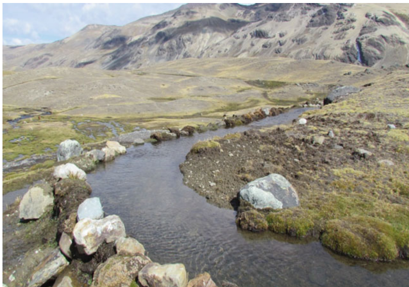
Photo 8 Start of the irrigation canal that transports water to grazing sites and small lagoons
