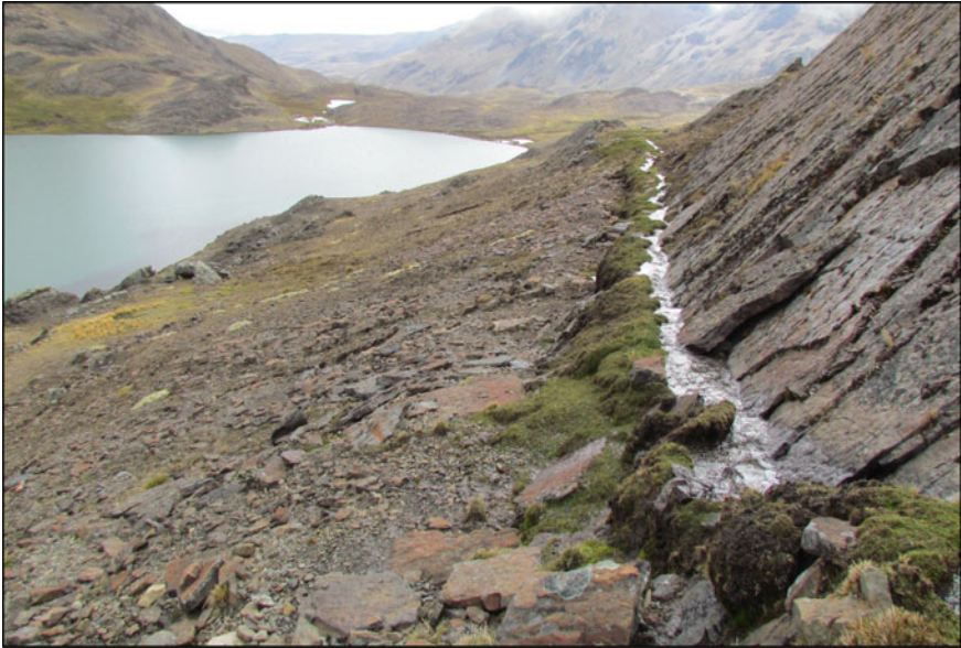
Photo 7 Local bioengineering work showing the path of the irrigation canal with Khuli tepes on a rocky hillside
