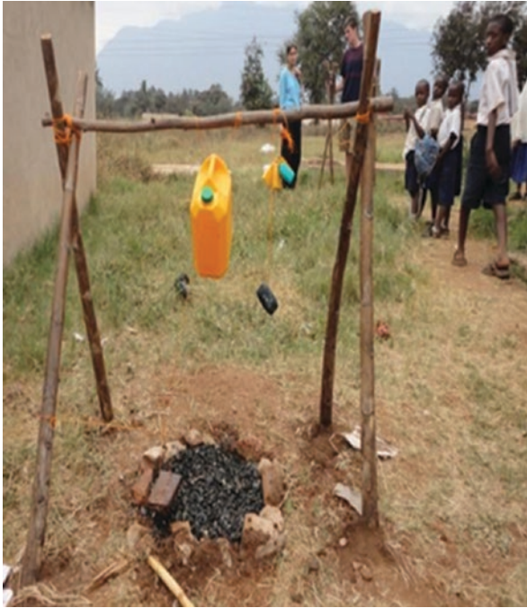
Fig. 24.3 A “tippy tap”—the foot pedal (lower left) would tilt the can so water comes out without having the user touch the can. Used water runs through a charcoal patch on the ground which absorbs/eliminates pathogens and toxins while the water is draining into the ground. If the can would be a transparent one, UV light would provide additional sterilization. Instead of a cap you could use a clean hose similar to one for petrol cans that makes the water run out more smoothly. The next step of invention would be a unidirectional valve that would prevent anything from entering the can—that would obviate the necessity for having to remove and put back the lid with the (contaminated) hand! (Photo and description courtesy of Chris Harkensee)
