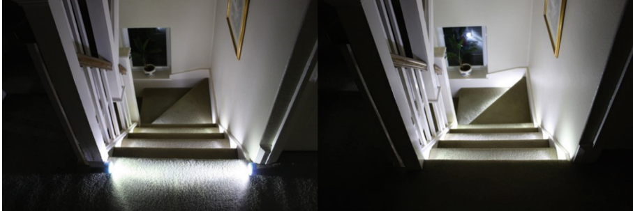
a) Localised LEDs on a domestic stair
