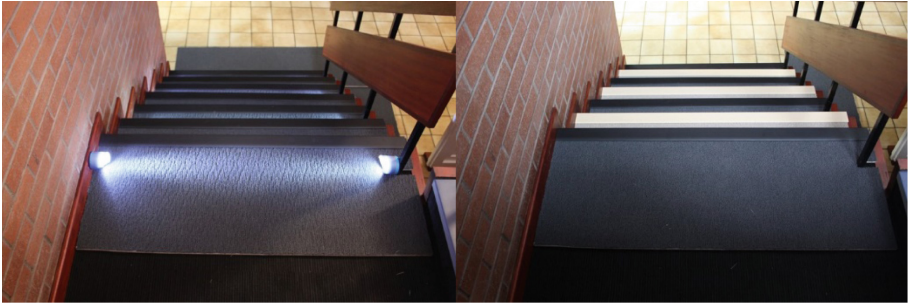
a) Localised LEDs and nosings on carpet
