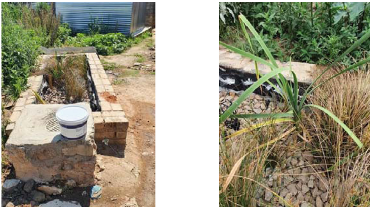
Fig. 3. Adaptation to the water collection system where the constructed wetland was used as a “table” (left) and adaptation to the constructed wetland ecosystem with new plant species arising spontaneously (right).
